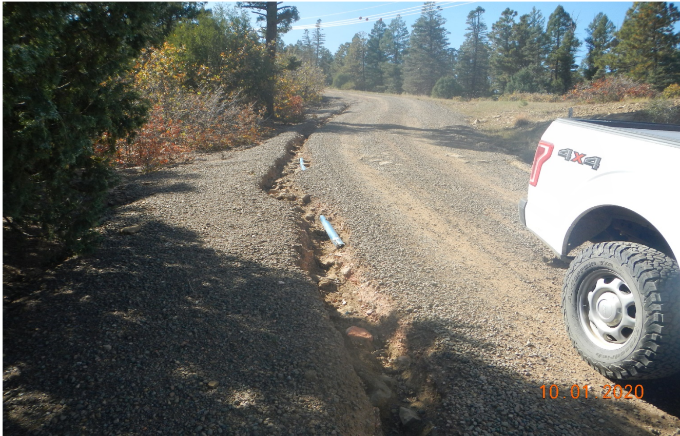
Photo 4. An eroaion channel has form along the steep grade of the road. Stormwater needs to be properly diverted and BMP's need to be installed. E.G Water bars, Sediment trap, check dams.
