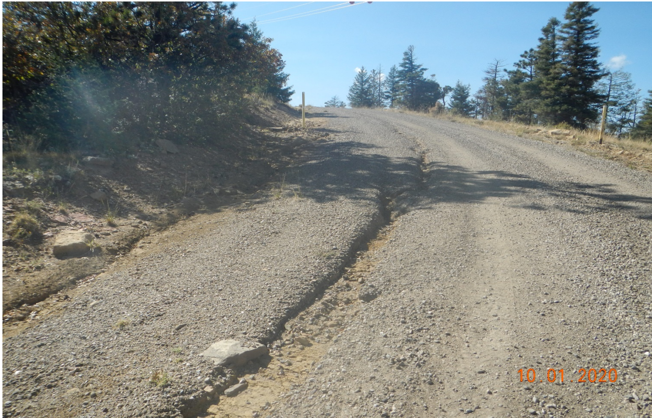
Photo 6. An erosion channel has formed along the steep grade of the road. Stormwater needs to be properly diverted and BMP's need to be installed. E.G Water bars, Sediment trap, check dams.
