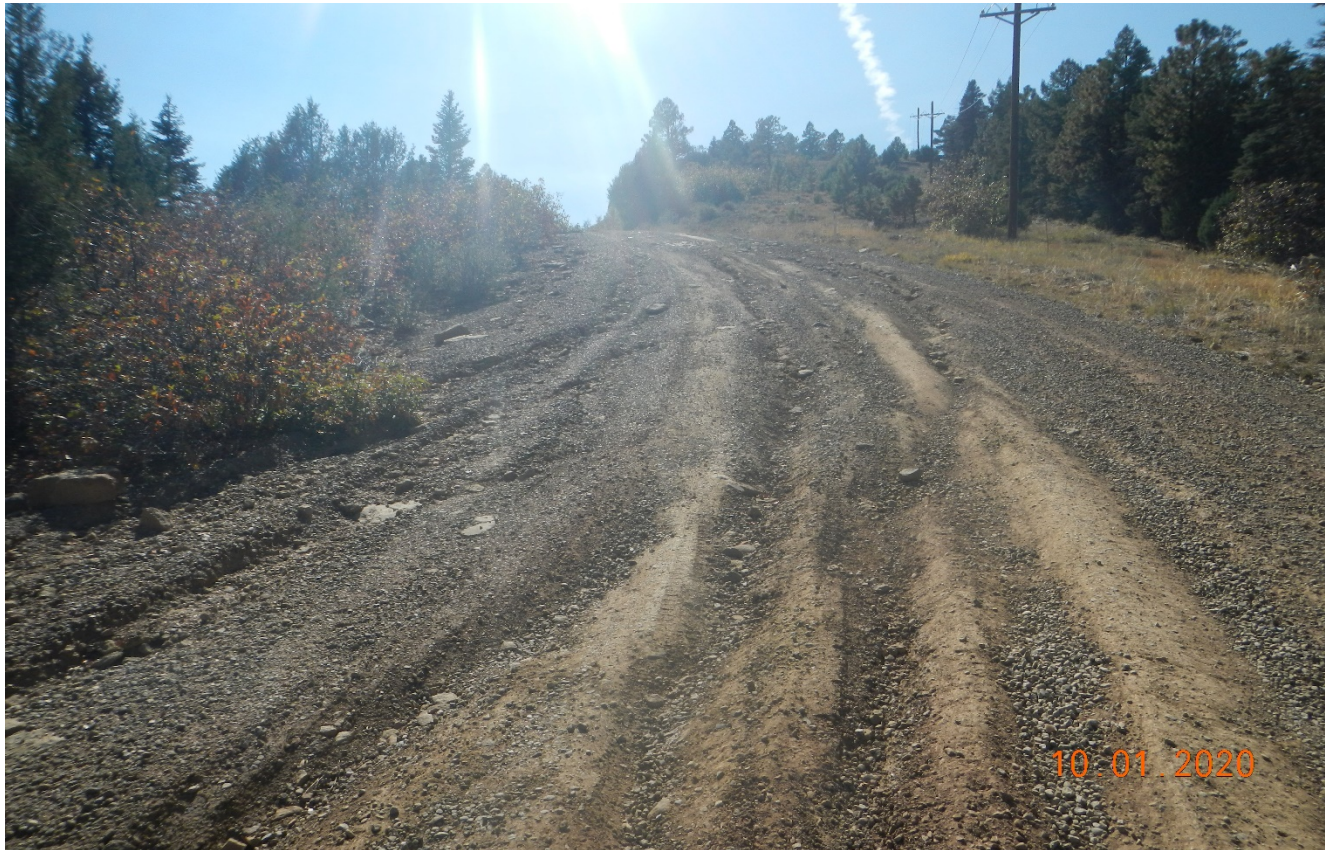
Photo 3. Facing west along the road. There is signs of erosion occurring down the road. BMP's need to be installed to prevent erosion and degradation of the road. E.G. Water bars.
