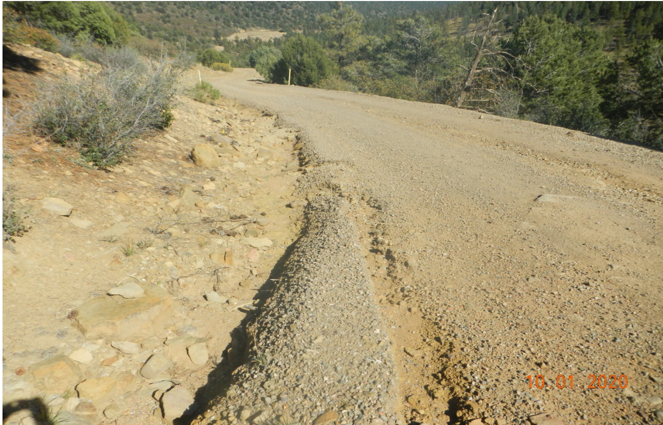
Photo 5. Stormwater is flowing down the road which is causing erosion and degradation of the road.
