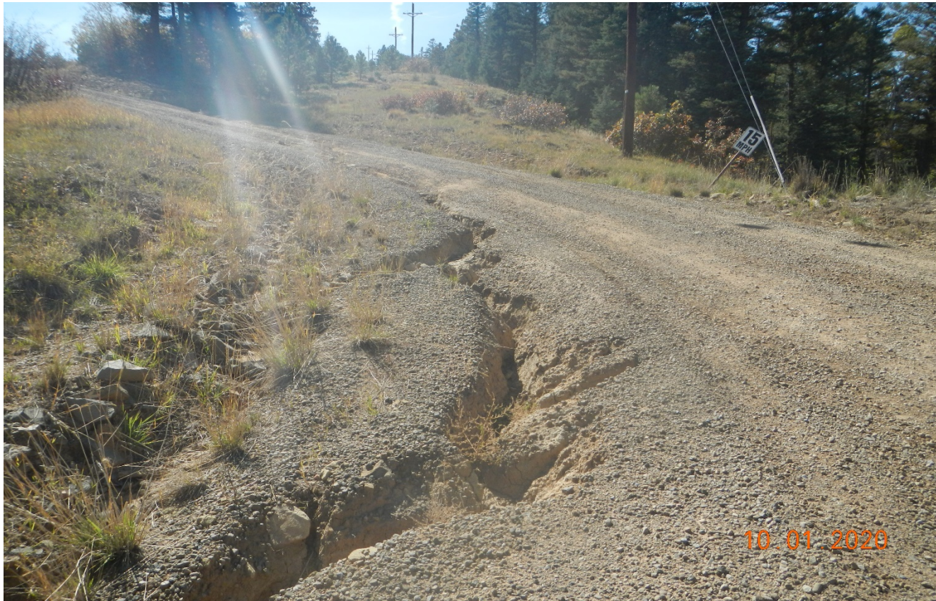
Photo 2. There is erosion that has occurred along the road ascending the hillside. Erosion needs to be repaired and BMP's need to be installed.
