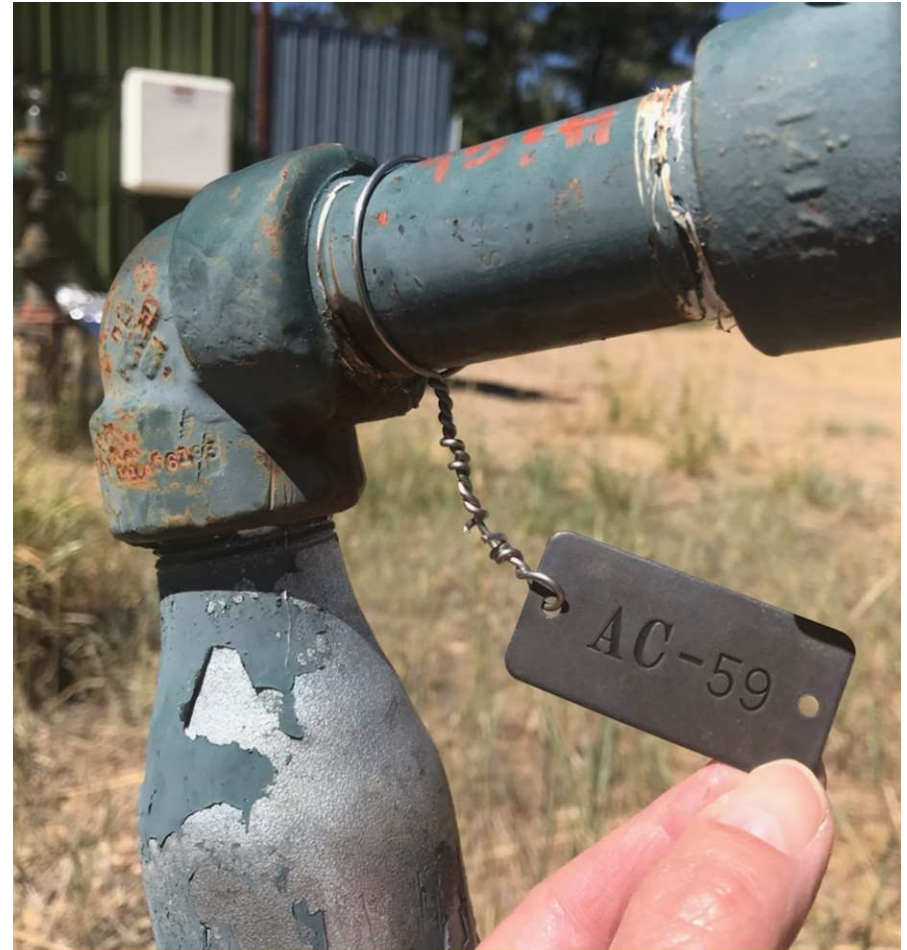
PHOTO 1: THE (2) RISERS ARE IN USE AND EACH ONE HAS BRASS TAG WHICH ARE VISABLE IN THE FIELD INSPECTION REPORT DOC # 695103256 PHOTO # 3 DOC # 695103260. THE NUMBERING SYSTEM IS STAMPED ON IT TO IDENTIFY THE DRIP RISERS. AC-58 AND AC-59 ARE ABBREVIATED FOR APACHE CANYON DRIP # 58 AND APACHE CANYON DRIP # 59.
