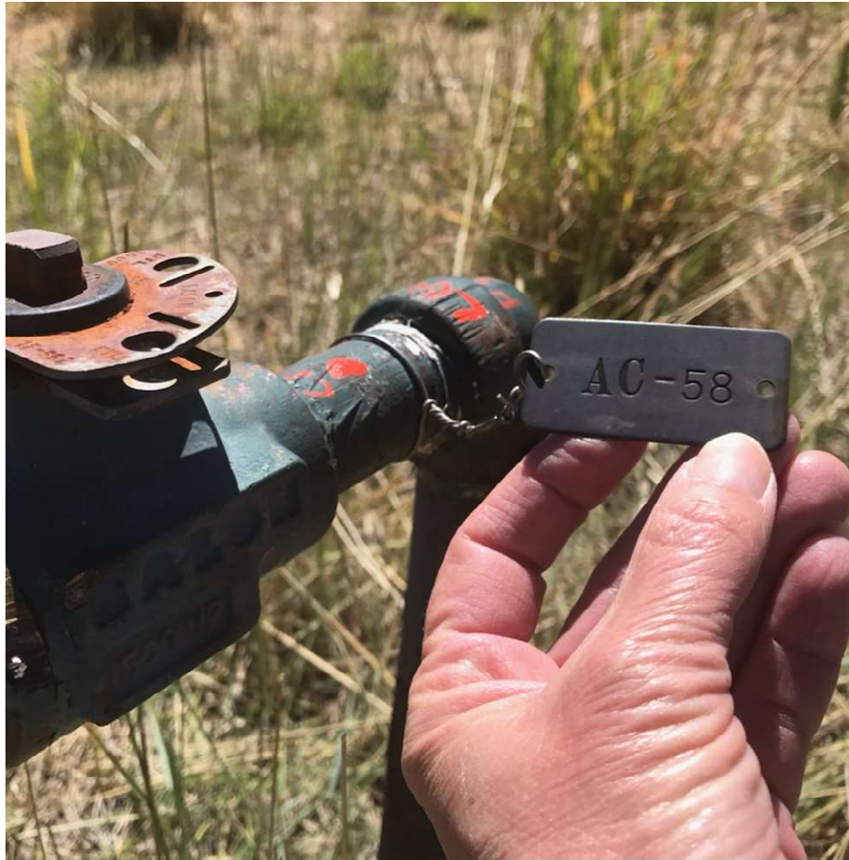
PHOTO 1: THE (2) RISERS ARE IN USE AND EACH ONE HAS BRASS TAG WHICH ARE VISABLE IN THE FIELD INSPECTION REPORT DOC # 695103256 PHOTO # 3 DOC # 695103260. THE NUMBERING SYSTEM IS STAMPED ON IT TO IDENTIFY THE DRIP RISERS. AC-58 AND AC-59 ARE ABBREVIATED FOR APACHE CANYON DRIP # 58 AND APACHE CANYON DRIP # 59.
