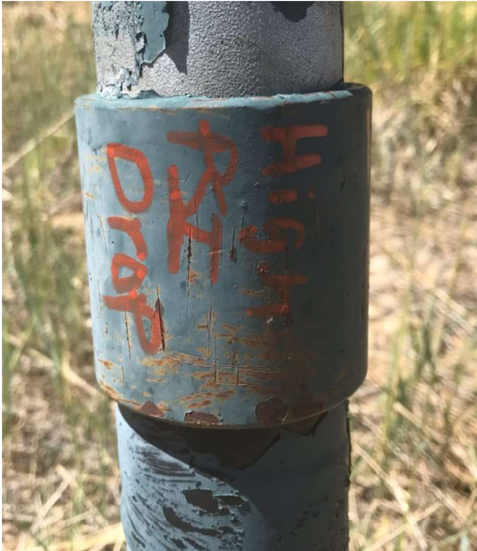
PHOTO 2: THERE IS A HIGH PRESSURE DRIP RISER AND A LOW PRESSURE DRIP RISER THAT ARE IN USE AND WERE MARKED WITH AN ORANGE MARKING PIN FOR ADDITIONAL IDENTIFICATION.
