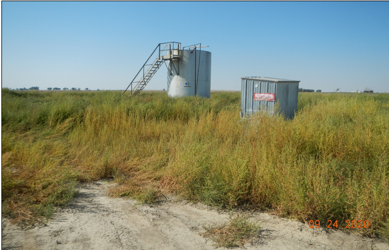
Photo 5. Facing southwest at the location. The meter shed and tank battery remains. All equipment should have been removed within 3 months of abandonment.
