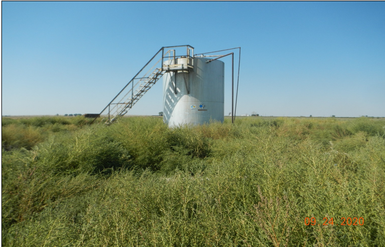
Photo 7. Facing toward the tank battery. The weeds are thick and overgrown that the surface of the location was not visible. It is unknown if there is secondary containment.
