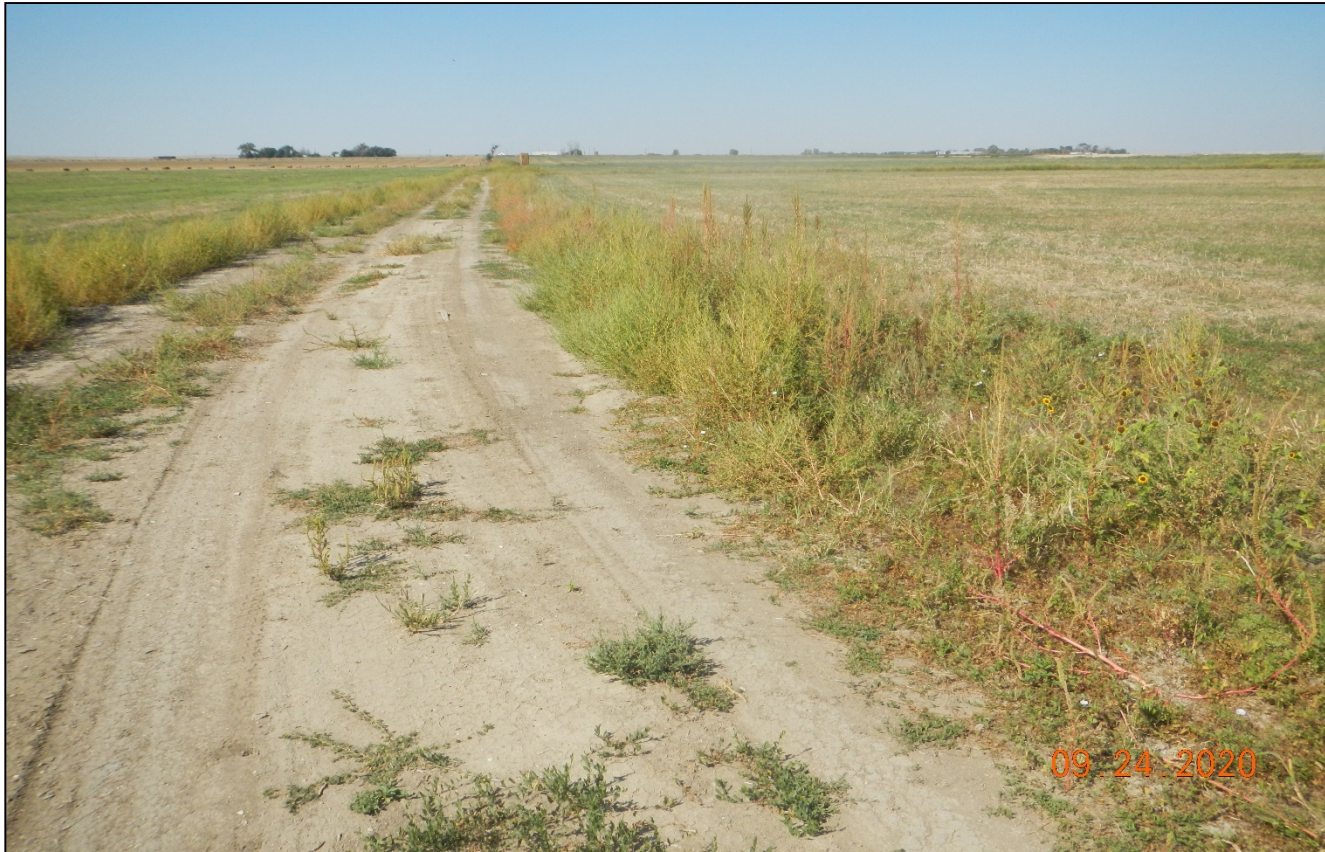
Photo 1. Facing west along the access road. The access road has not been reclaimed and there is undesirable weeds along the roadside.
