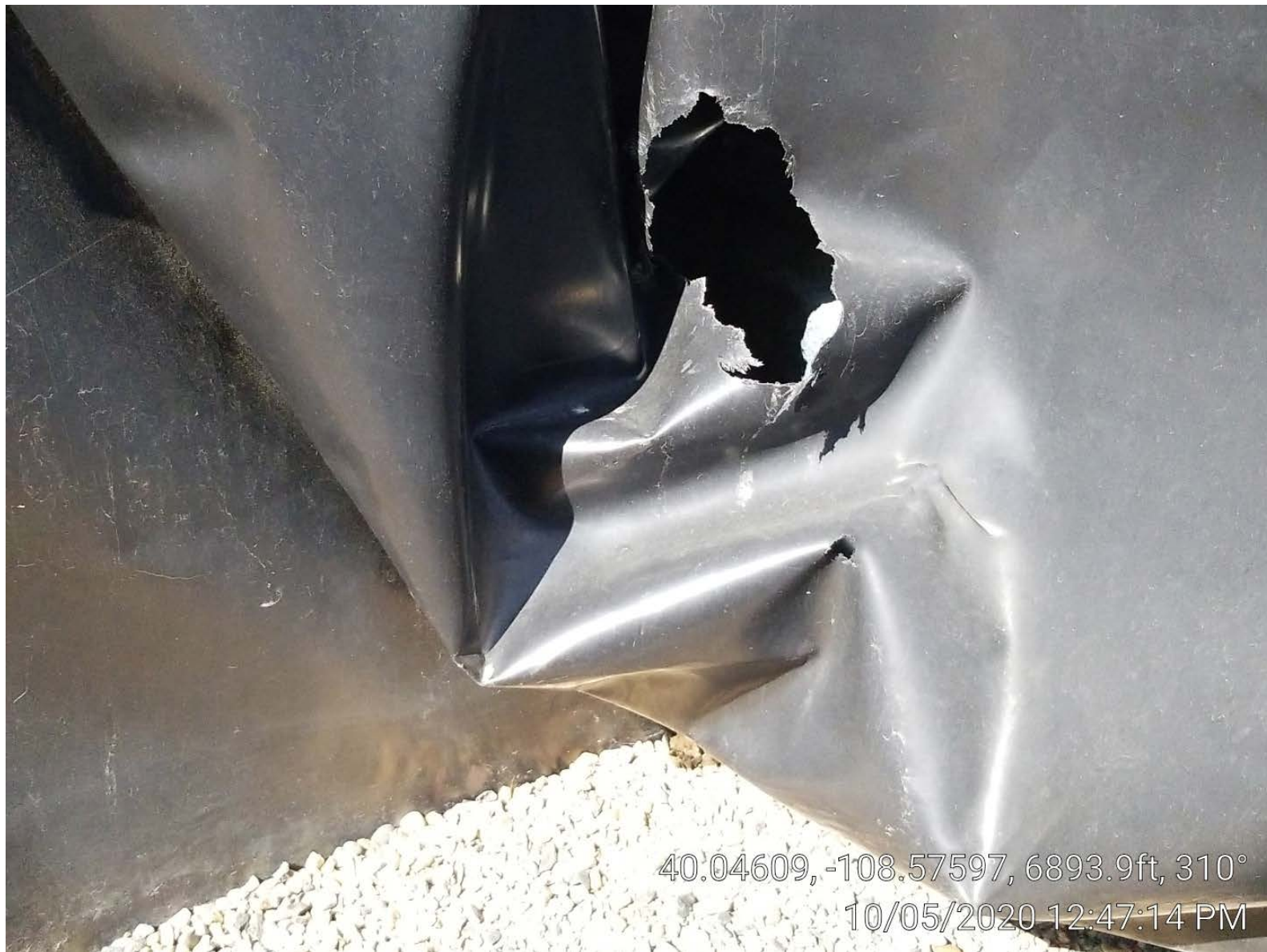
Photo 5. Tank secondary containment liner.
