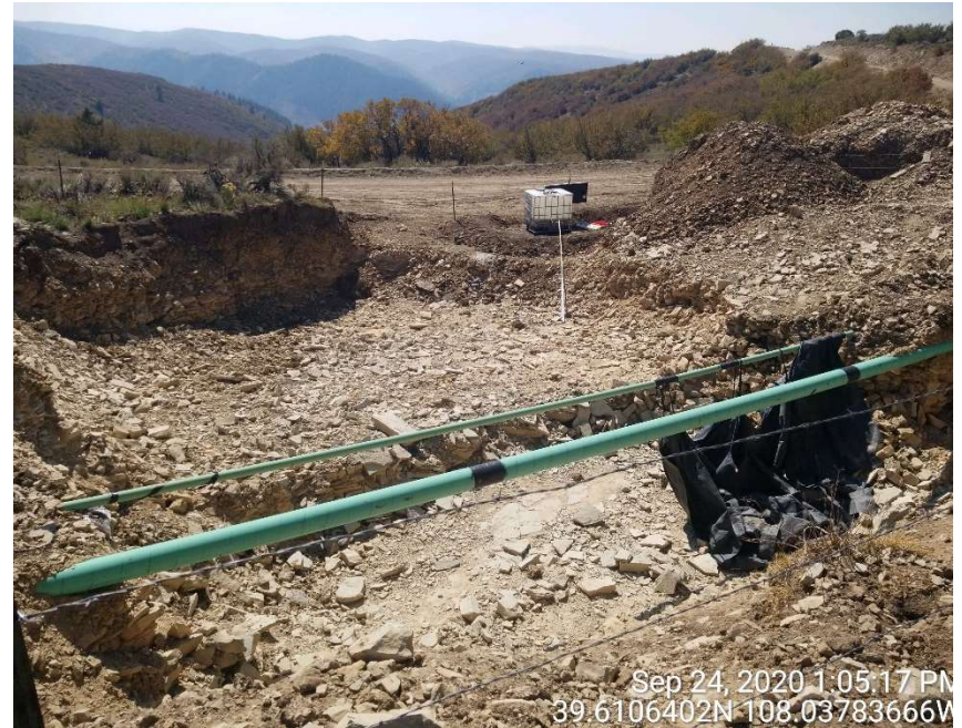
Spill/release area excavation.
