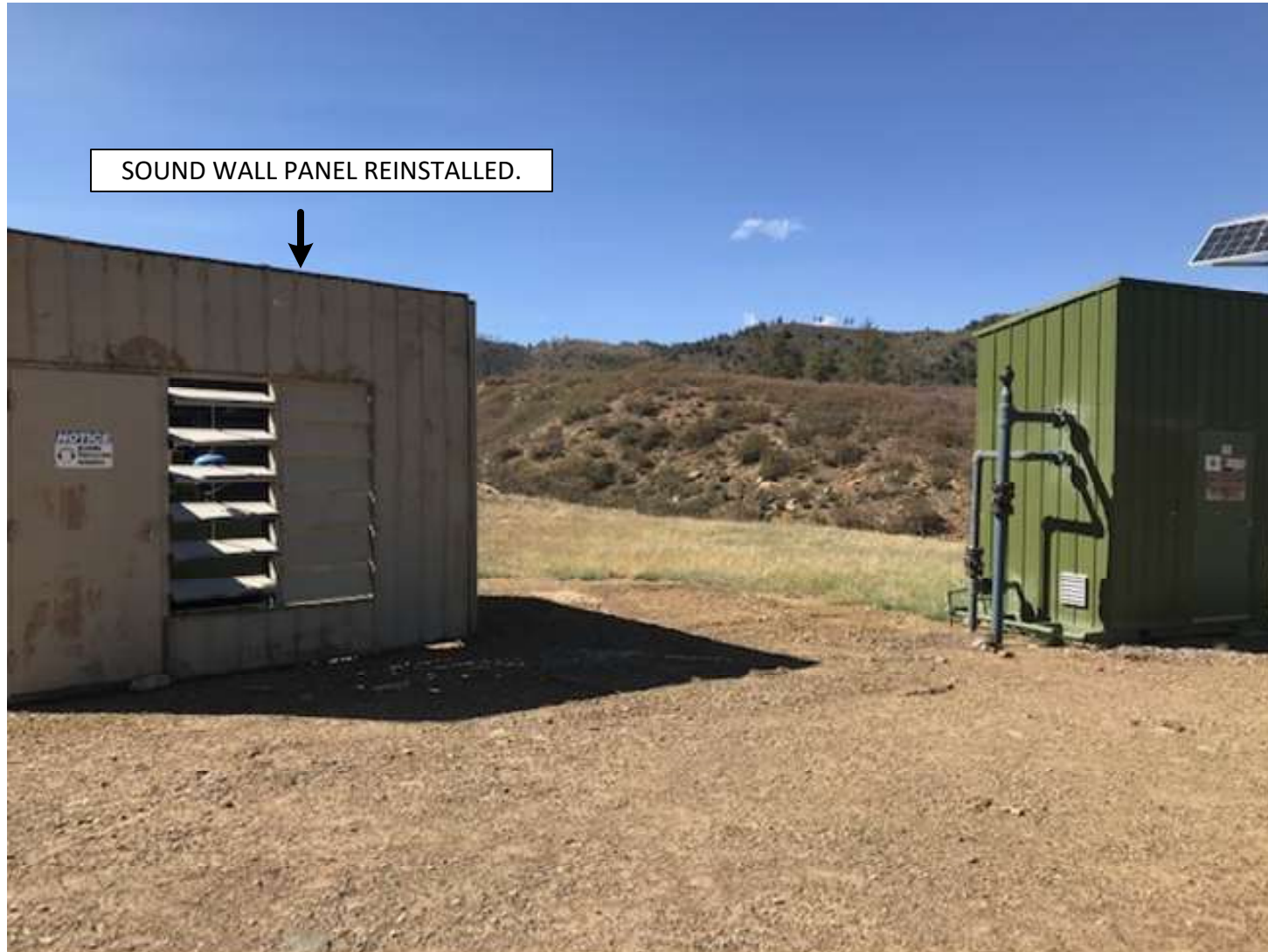
PHOTO 2: THE SOUND WALL PANEL THAT WAS ON THE GROUND WAS REINSTALLED SURROUNDING THE ENGINE SKID.
