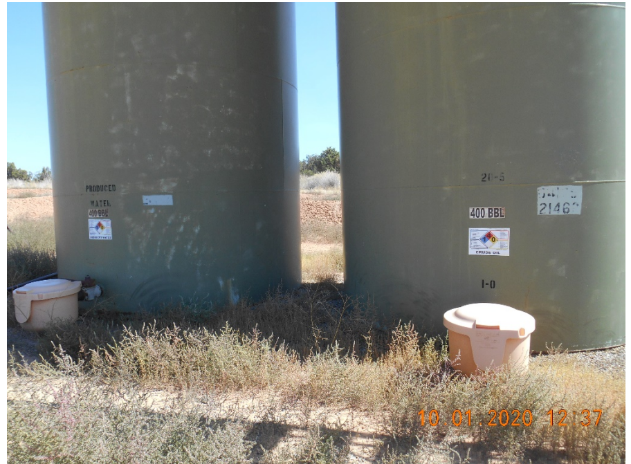
Tank Battery with improper tank labels.
