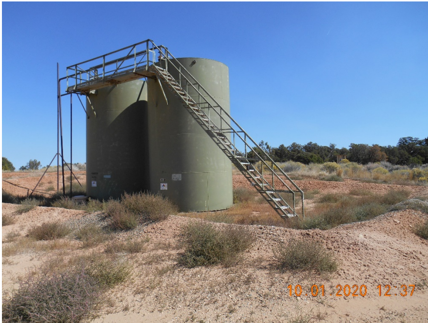
Tank Battery with earth berms. Weeds inside berms.
