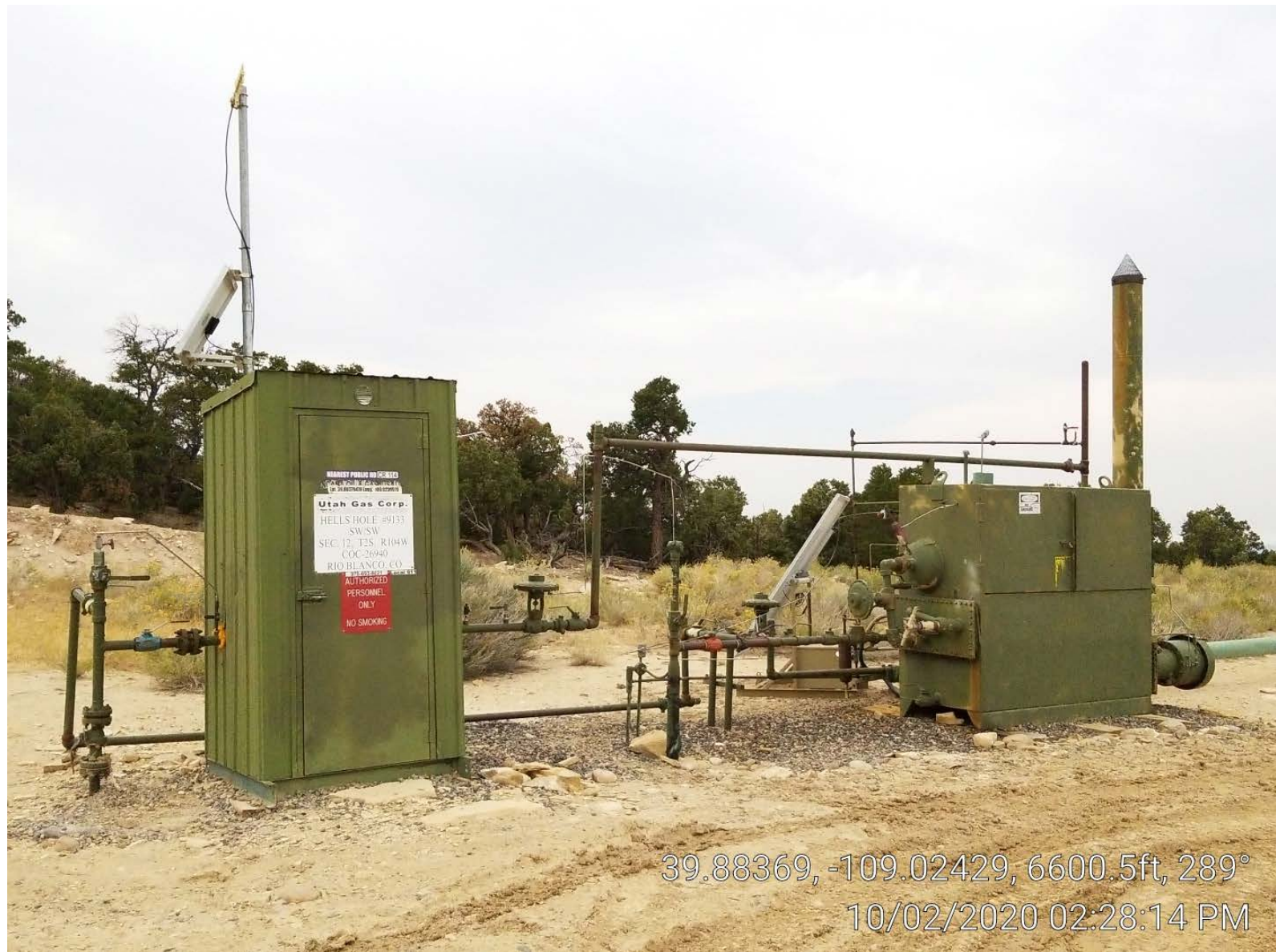
Photo 6. Meter building & separator.
