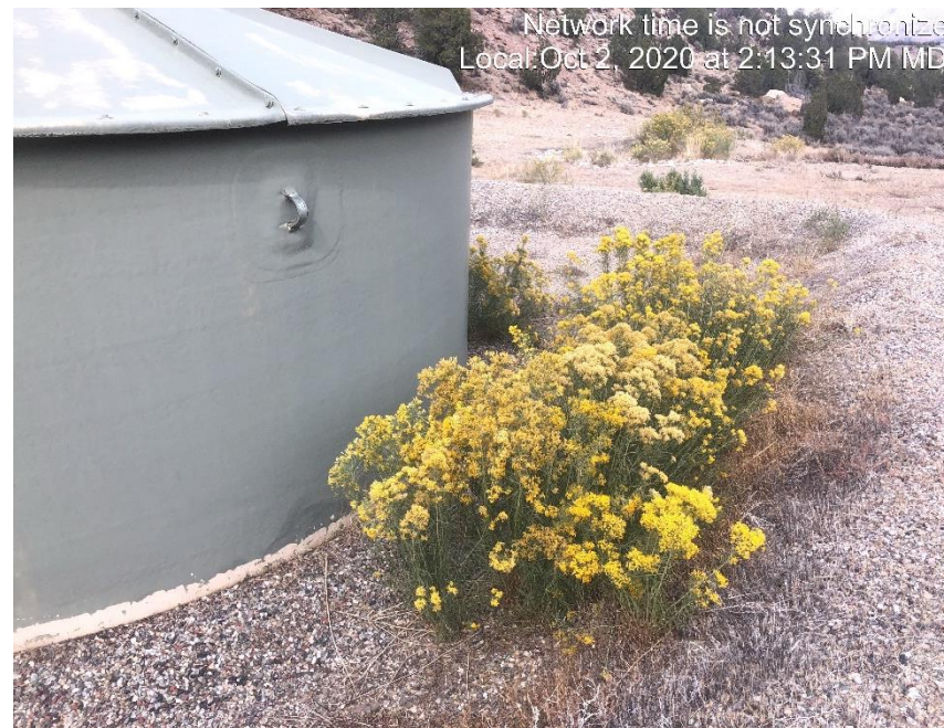
Photo 31977 Secondary containment not adequate weeds growing inside tank containment.
