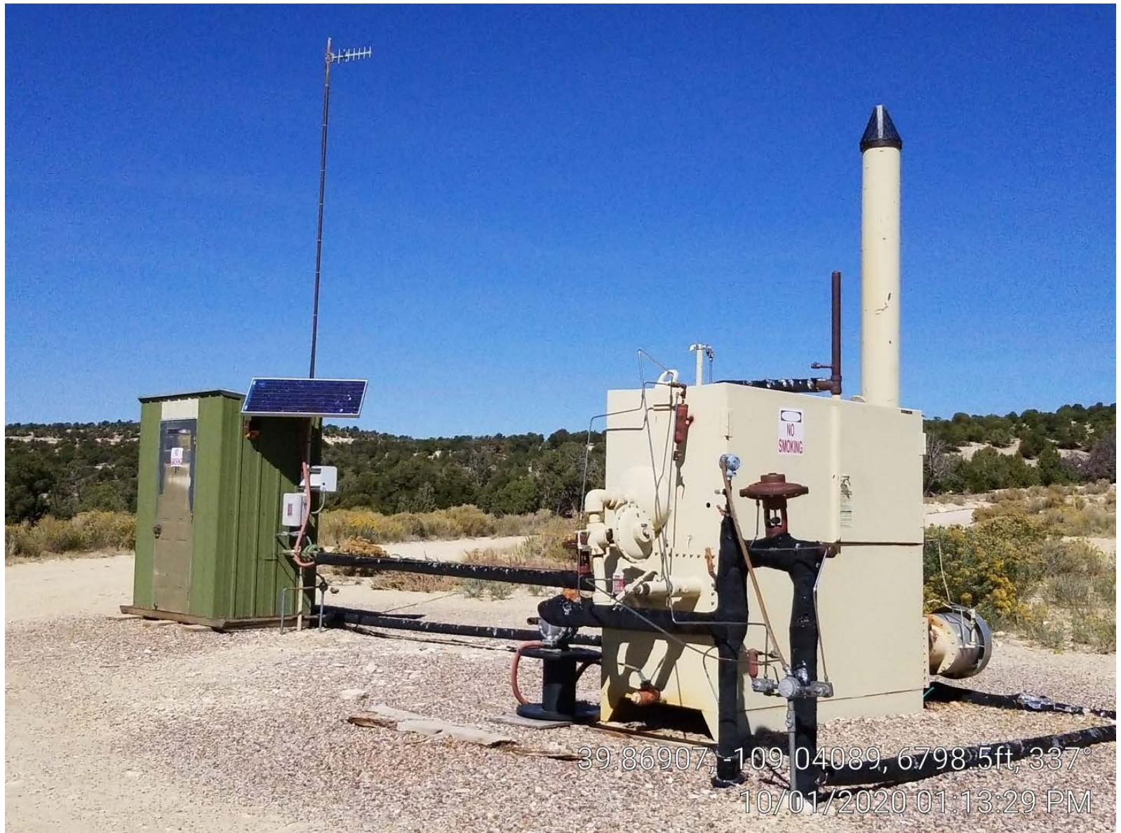
Photo 3. Meter building & separator.
