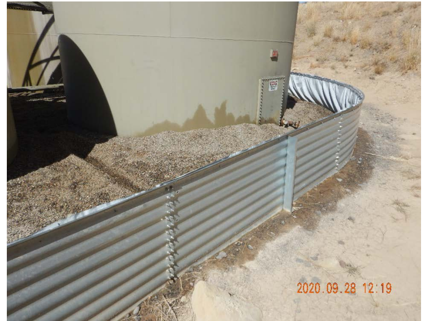
Photo #10 - View of impacted soil outside of secondary containment ring along northeast side of tank battery.
