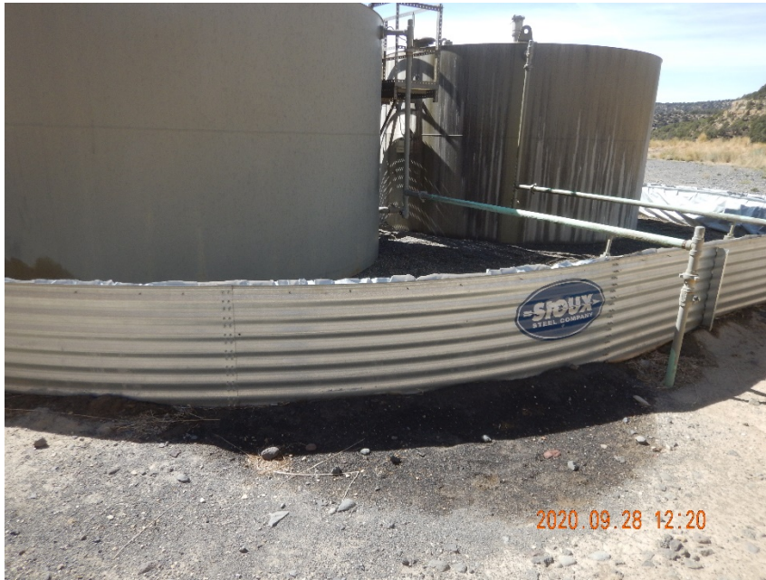
Photo #7 - View of impacted soil outside of secondary containment ring along northeast side of tank battery.
