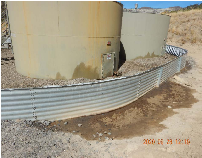
Photo #9 - View of impacted soil outside of secondary containment ring along east side of tank battery.
