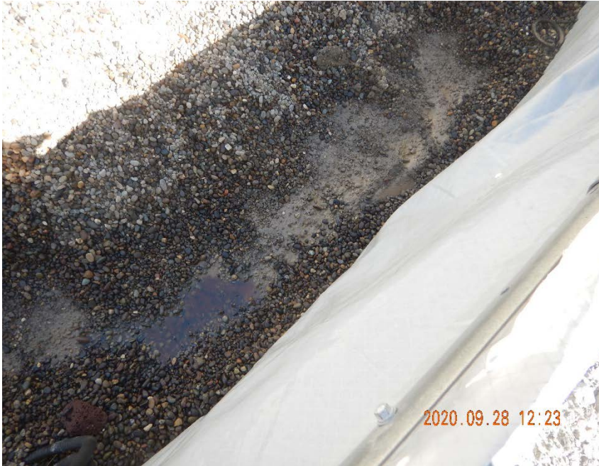
Photo #13 – Hydrocarbon-impacted gravel and fluids remaining inside of tank battery secondary containment (south side).
