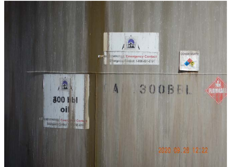
Photo #16 – Tank labels and NFPA placard on northwest condensate AST, note conflicting volume labels.
