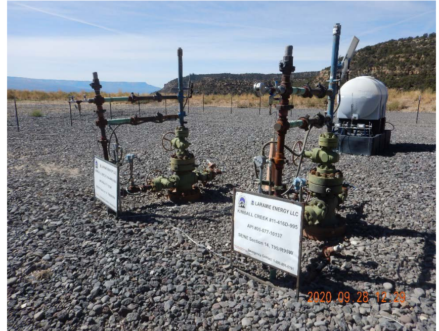
Photo #18 – Wellheads located ~120 feet southwest of tank battery.
