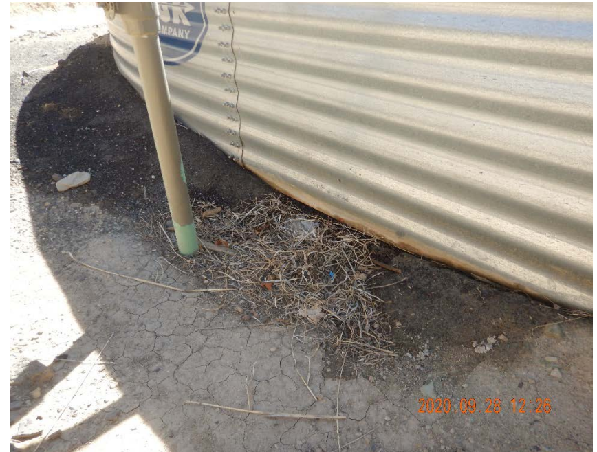
Photo #8 – Impacted soil at flowline riser on north side of tank battery.
