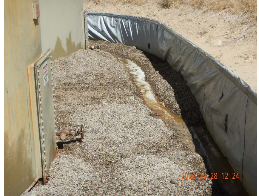
Photo #14 - Hydrocarbon-impacted gravel and fluids remaining inside of tank battery secondary containment (east side).
