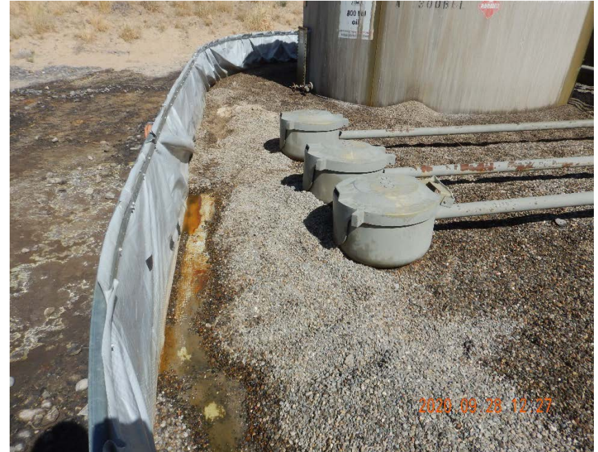
Photo #12 – View of loadout area on west side of tank battery. Tank battery secondary containment area contained hydrocarbon-impacted gravel and fluids on inspection date.
