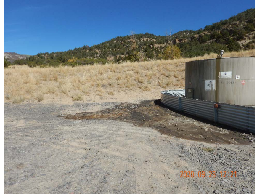
Photo #4 – Impacted soil outside of secondary containment ring located along west side of tank battery.
