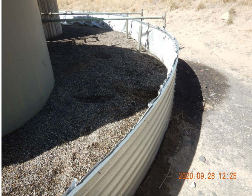
Photo #15 - Hydrocarbon-impacted gravel and fluids remaining inside of tank battery secondary containment (north side).
