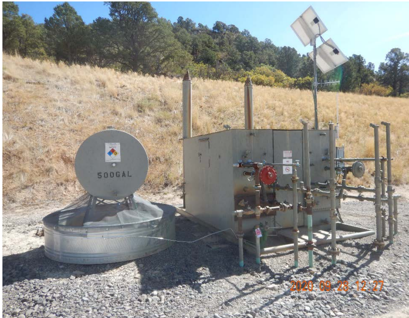
Photo #17 - Heated horizontal separators with 500 gallon methanol tank located ~75 feet southeast of tank battery.
