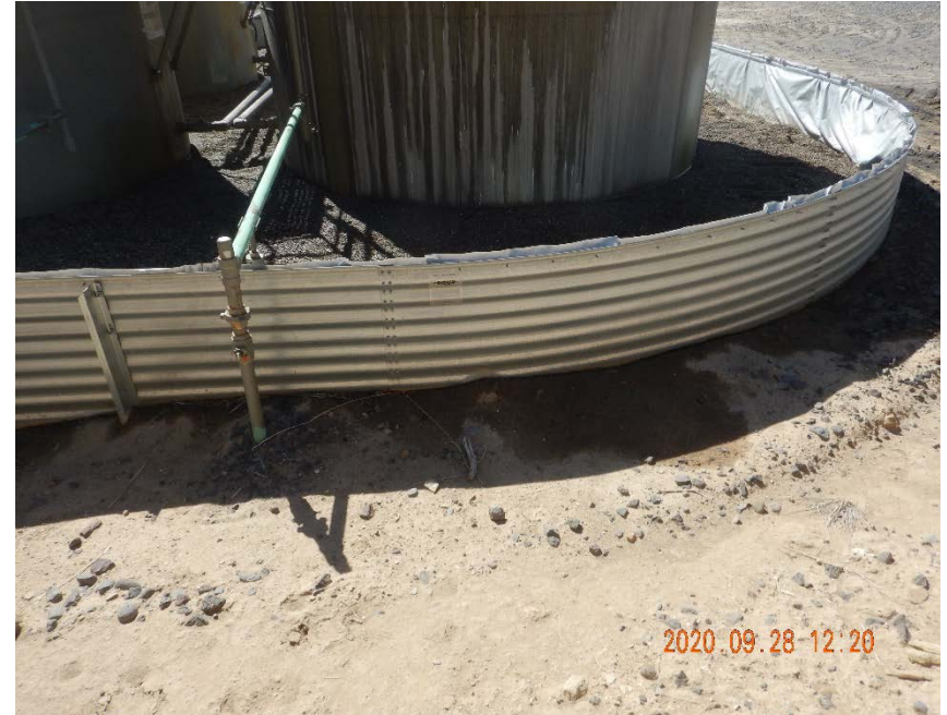
Photo #6 – View of impacted soil outside of secondary containment ring along northwest side of tank battery.
