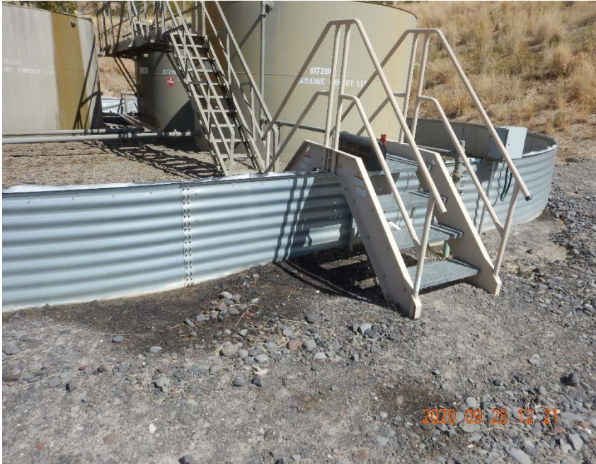
Photo #11 - View of impacted soil outside of secondary containment ring along south side of tank battery.
