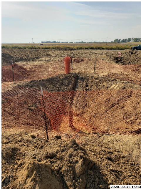
PICTURE OF MONFORT-BOSTROM 1 WELL - CAMERA ANGLE WEST
