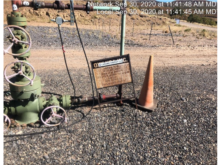
Photo #1956 Multiple wellhead signs weathered and not legible.
