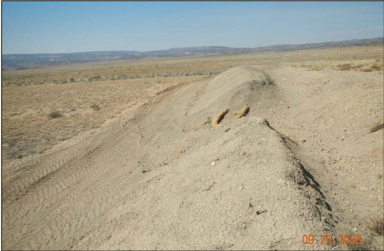
Photo 2. View of the stormwater controls installed and maintained in the southern project area.
