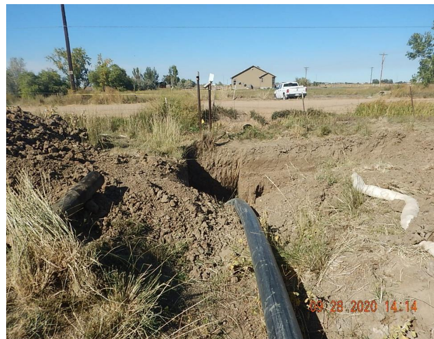
View from south excavation across WCR 4; looking north Replacement section of flowline being installed.
