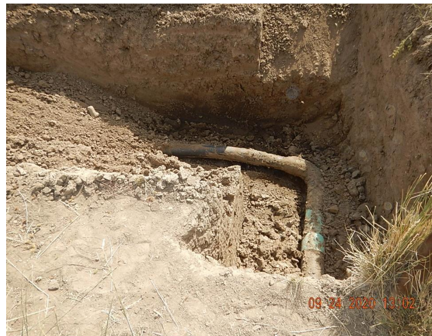
Close up view of flowline exposed in south excavation
