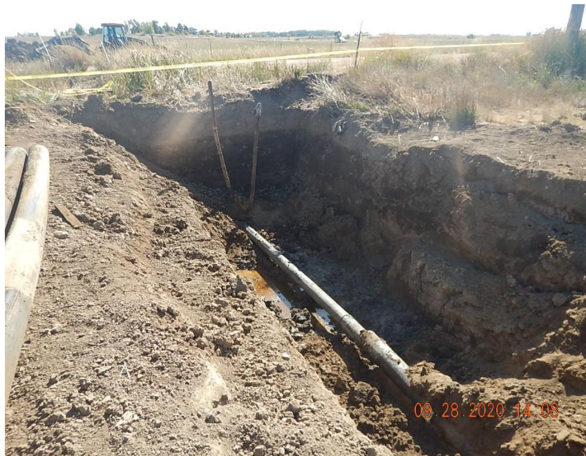
View of replacement section of flowline (new HDPE) that has been pulled under WCR 4 through casing pipe from south to north excavations.
