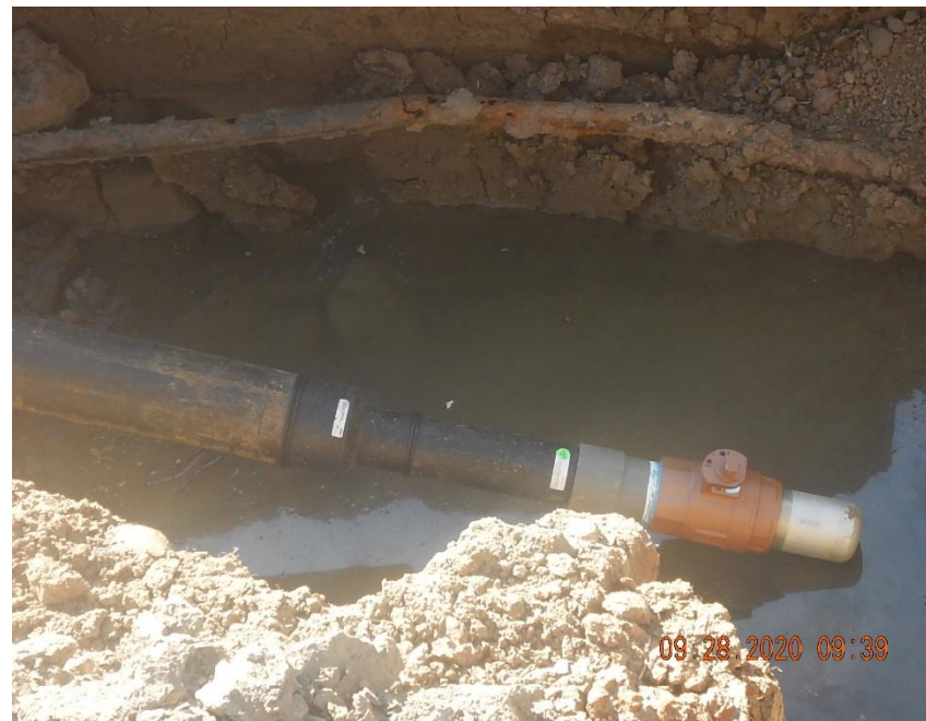
View of valve and bullplug installed at south excavation; Historically abandoned flowline also present in excavation.
