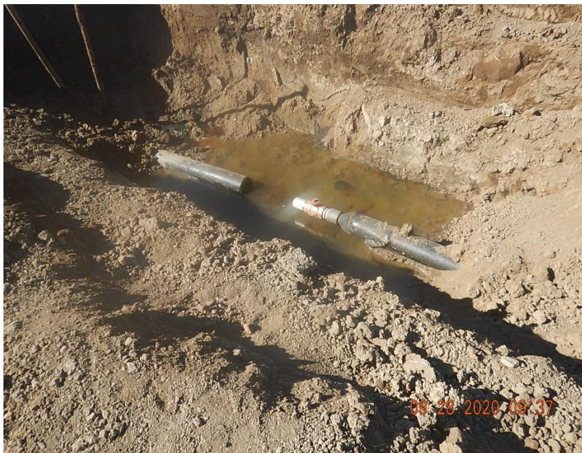
View of valve and bullplug installed at north excavation.
