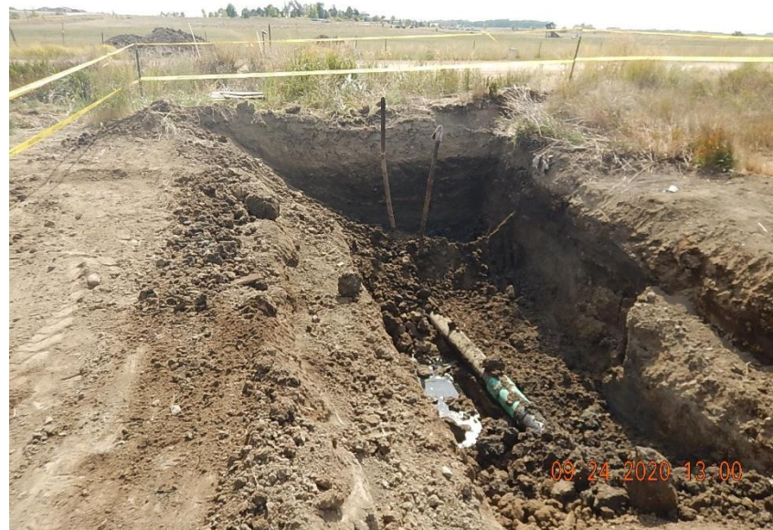
View of flowline exposed in excavation and pooled hydrocarbons; looking south.
