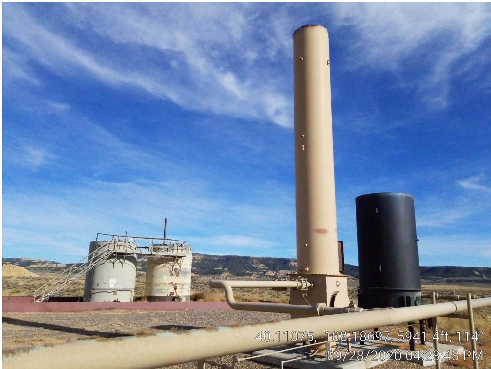
Photo 4. Emission control devices & tanks.
