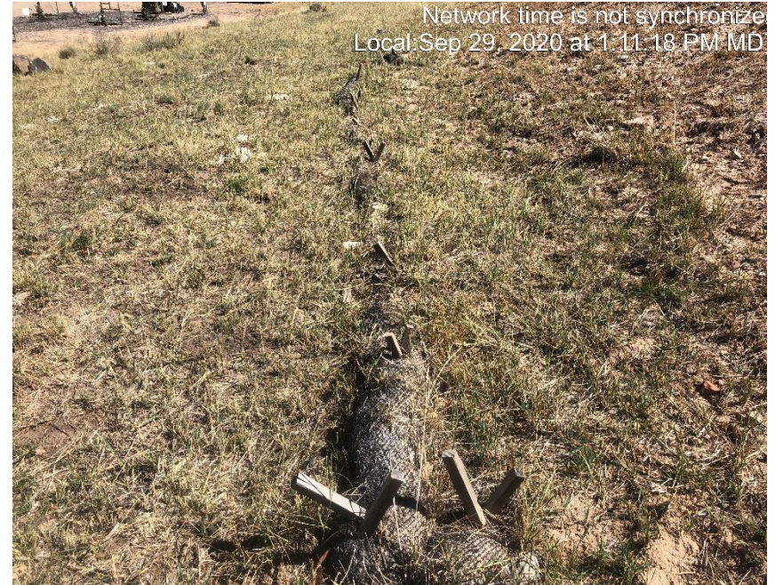
Photo #1947 Waddles on NW corner of the cut slope.
