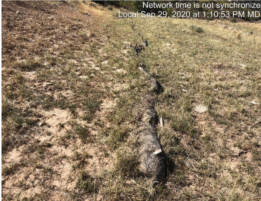
Photo #1946 Waddles on NW corner of the cut slope.
