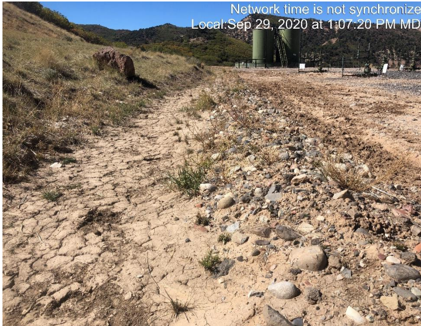
Photo #1944 Berm at base of SW cut slope.
