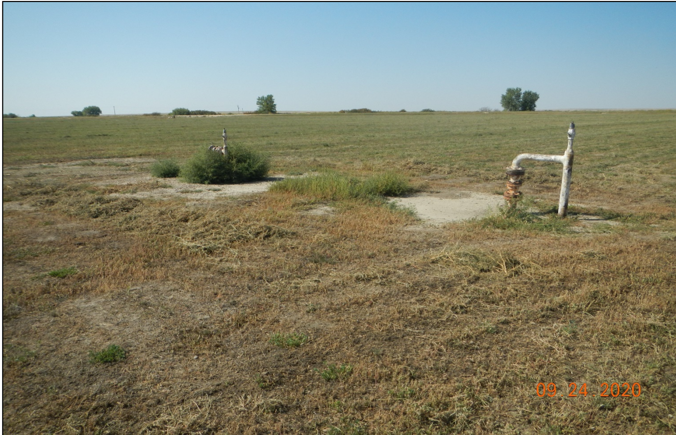
Photo 1. Facing southwest at the location. There are pipe risers that have not been removed and are interfering with farming operations.
