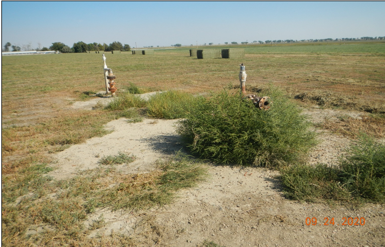
Photo 2. Facing northeast at the location. Abandoned risers need to be removed.
