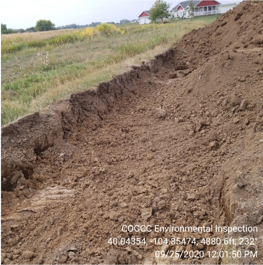
Photo 3 – Area of spill excavation
