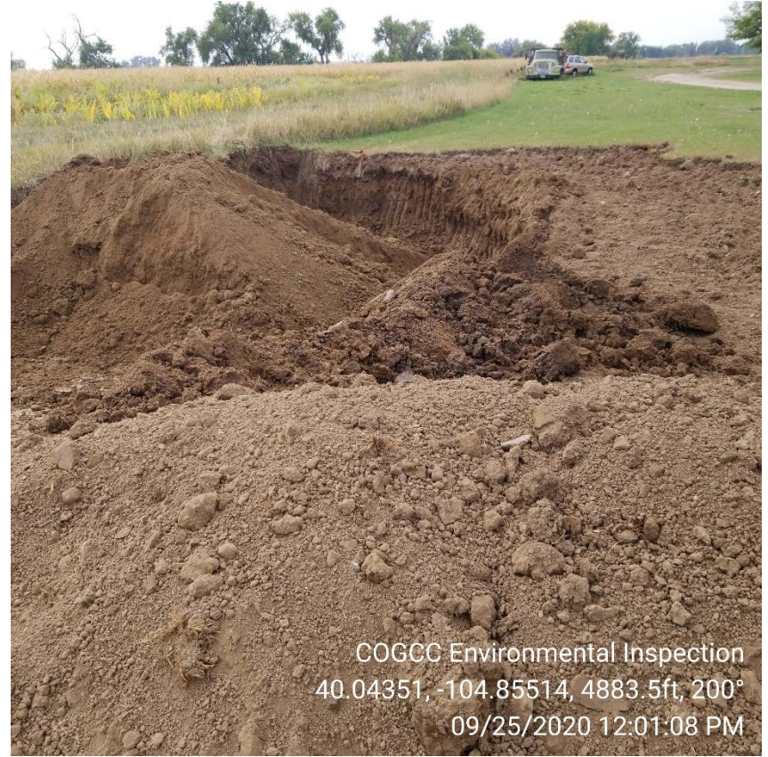
Photo 4 – Area of spill excavation
