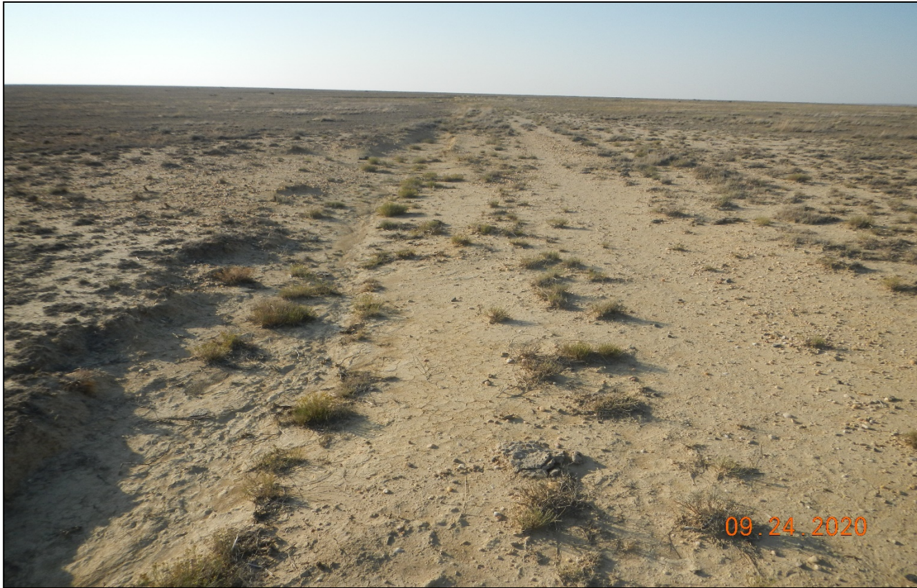
Photo 1. Facing south along the access road. There are signs of erosion along the road. The access road has not been reclaimed.
