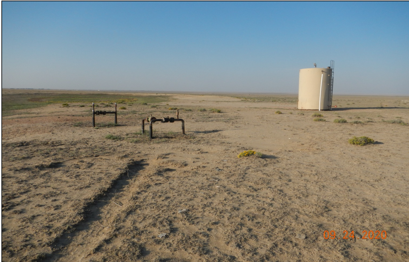
Photo 2. There is pipe risers that remain at the location and a steel tank. Does not appear to be in use. Unused equipment needs to be removed.
