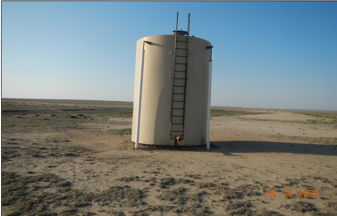
Photo 3. A steel tank appears to be unused with no secondary containment. There is no vegetation growth around the tank which indicates impacted soil.
