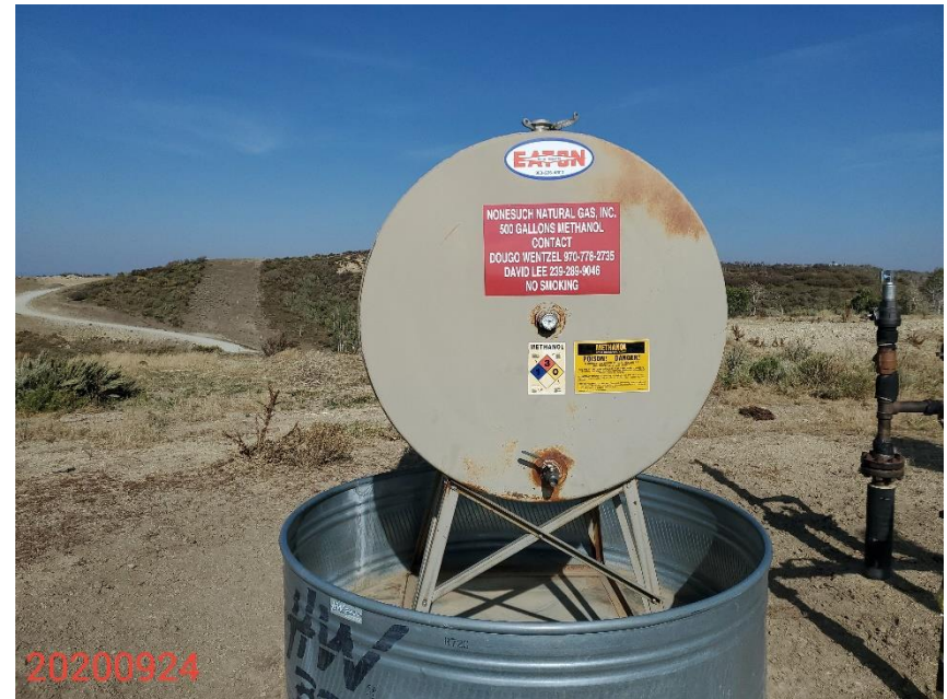
Photo 6: Photo shows methanol tank on the Location. It is unclear to the COGCC as to what the equipment's current use is on the Location, and if equipment is considered active.
