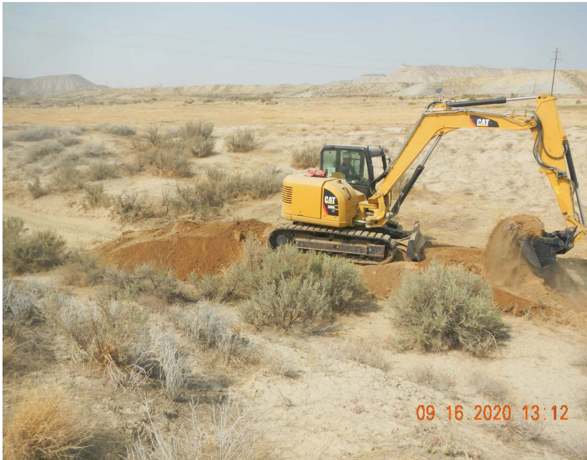
Photo #8 mini track hoe is further blending excavated soil and fill soil.
