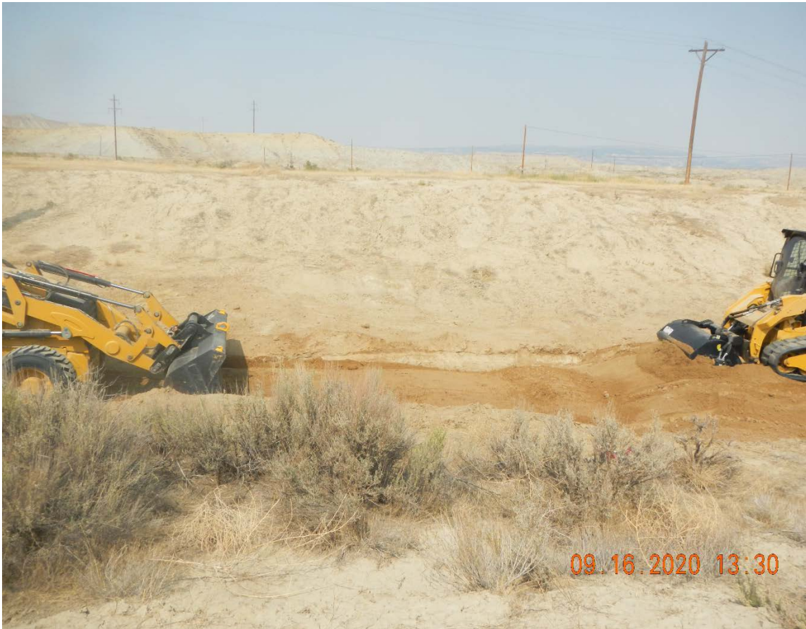
Photo #16 pushing in fill and tilling
