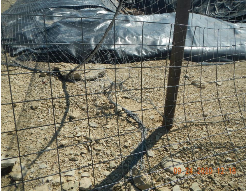
Gaps in fencing/netting around the pit in north west corner
