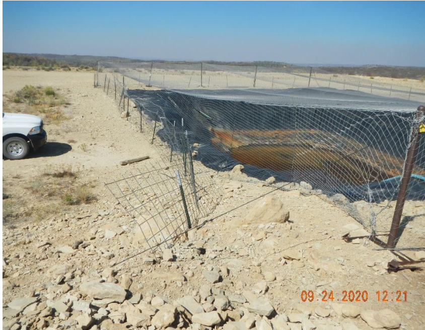
Gaps in fencing/netting around the pit in south east corner
