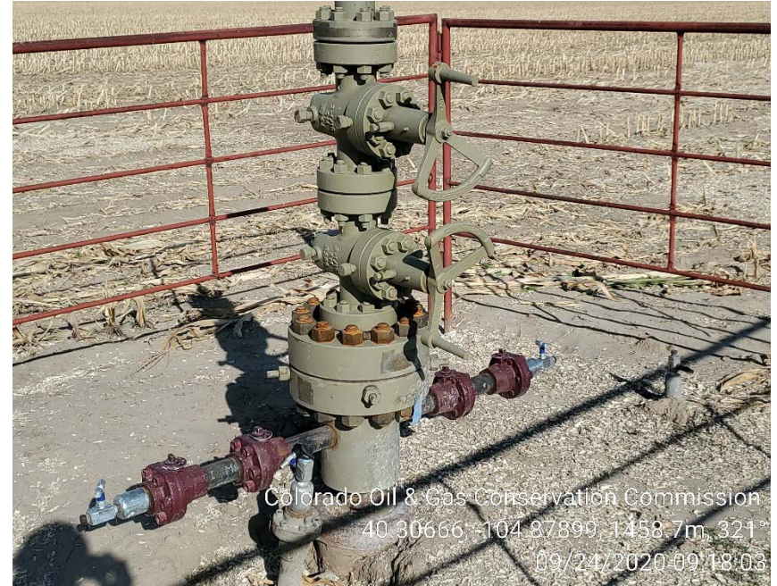
Wellhead and disconnected flowline
