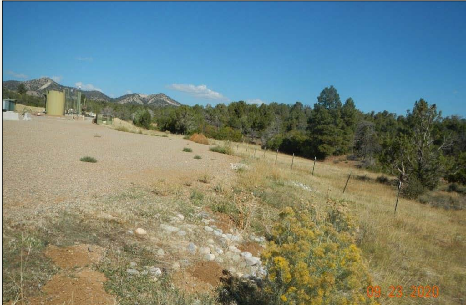
Photo 2. View of the eastern fill slope from the northeastern project area facing southward. Revegetation is progressing with grasses and shrubs such as western wheatgrass, rubber rabbitbrush, and sand dropseed.
