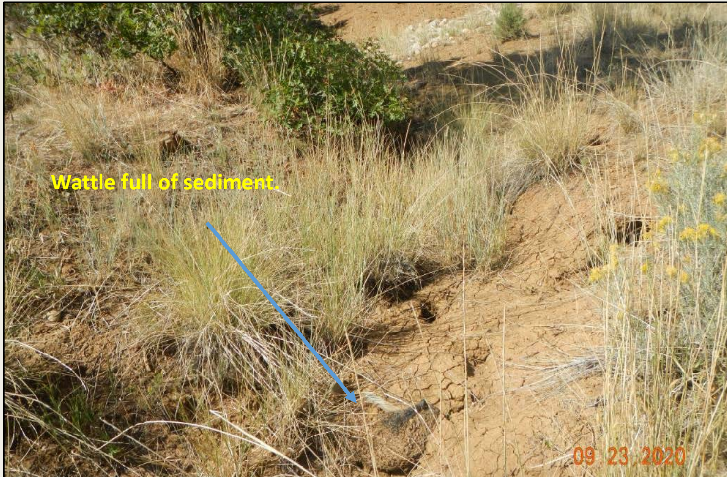
Photo 4. View of wattle in the drainage channel that is full of sediment and no longer functioning. BMP upstream of channel appears to be functioning at this time.
