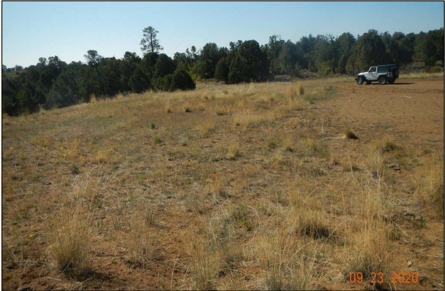
Photo 2. View of the southern fill slope from the southeastern edge facing westward. Revegetation is progressing with grasses such as western wheatgrass, crested wheatgrass, and intermediate wheatgrass.
