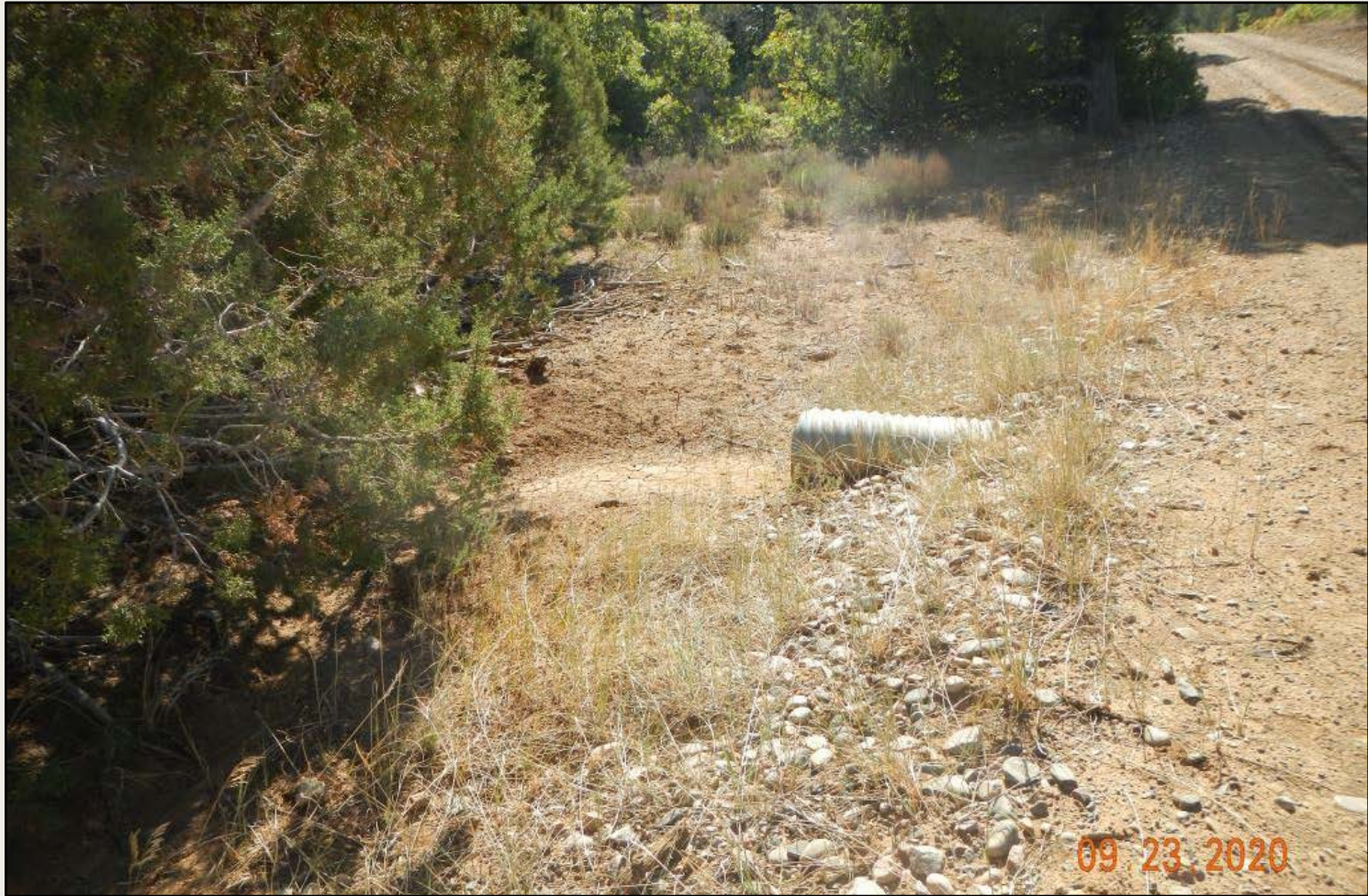
Photo 4. View of culvert outlet near the well pad entrance, appears to be stabilized at this time.
