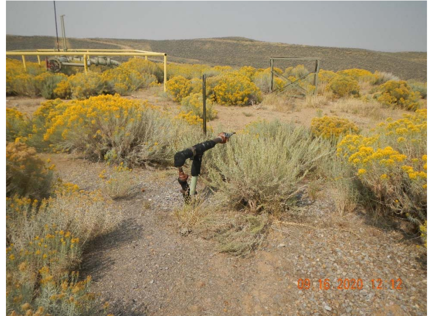
Photo 6. Riser not marked for LOT or abandonment.
