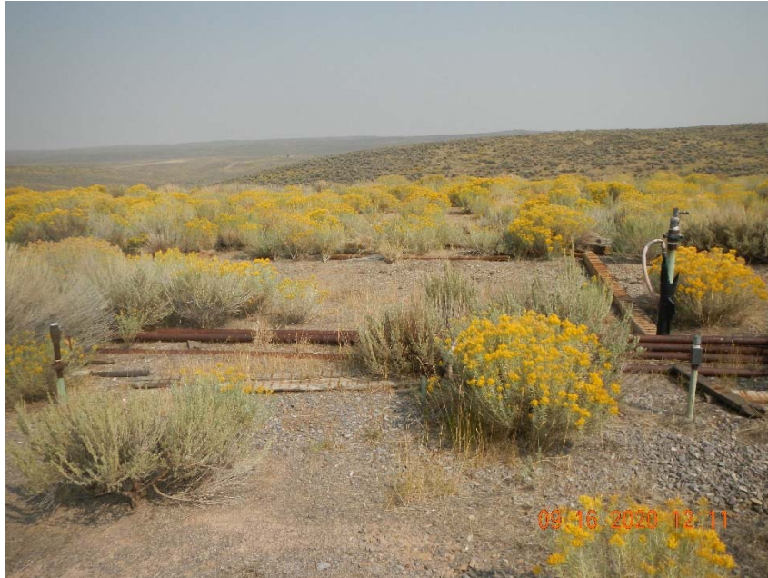
Photo 5. Risers not marked for LOTO or abandonment.
