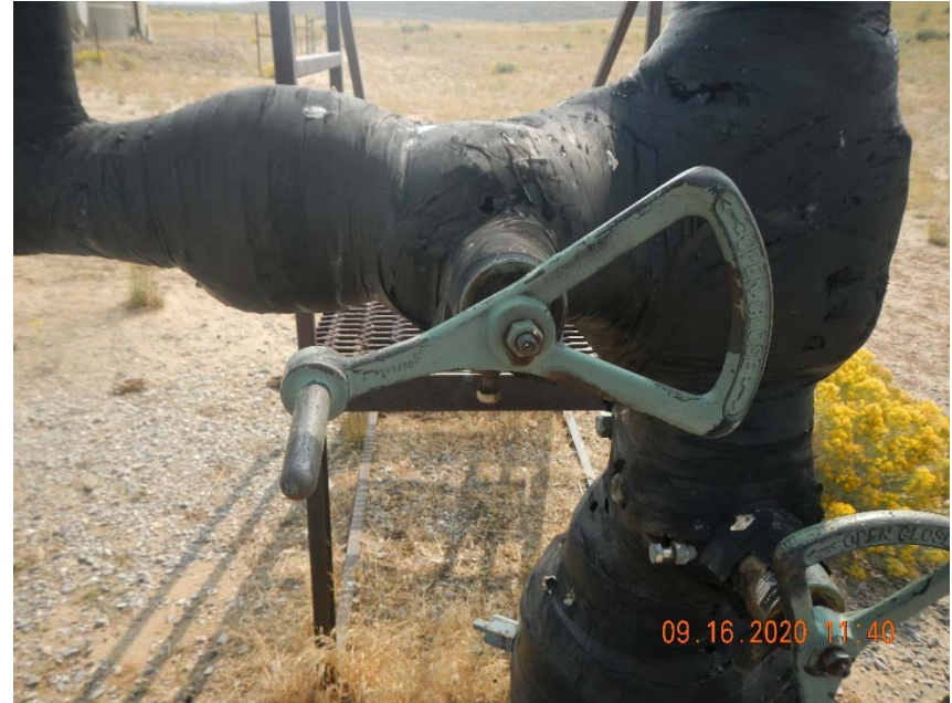
Photo 4. Hissing sound coming from this valve on wellhead.
