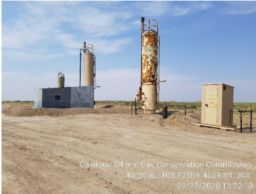
Photo 3 – Heater Treaters, Gas Meter
