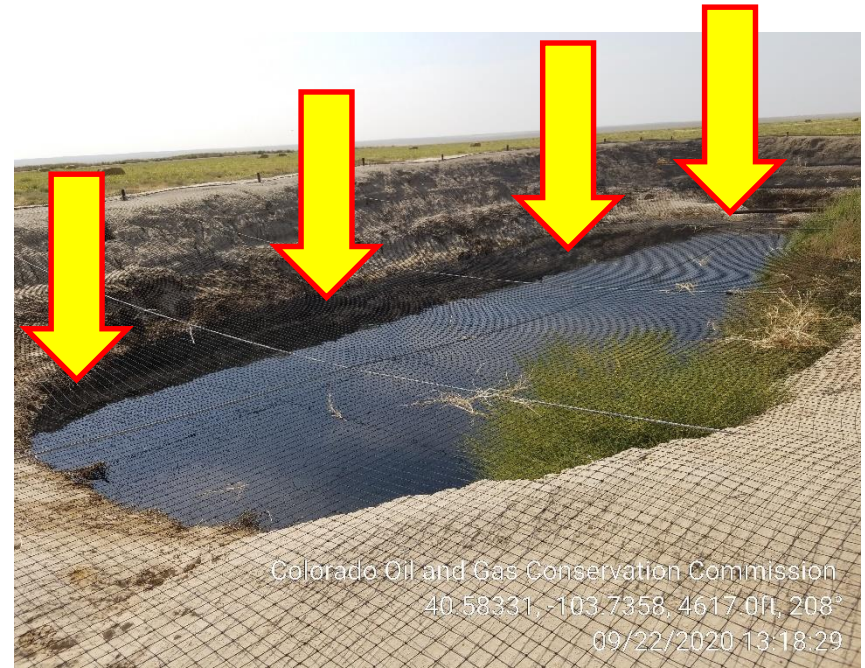
Photo 12 – Oil/Hydrocarbon on Pit. Stained Soil on the Edges
