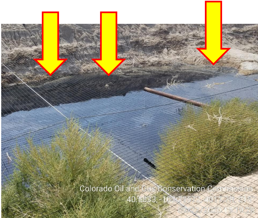
Photo 11 – Oil/Hydrocarbon on Pit. Stained Soil on the Edges
