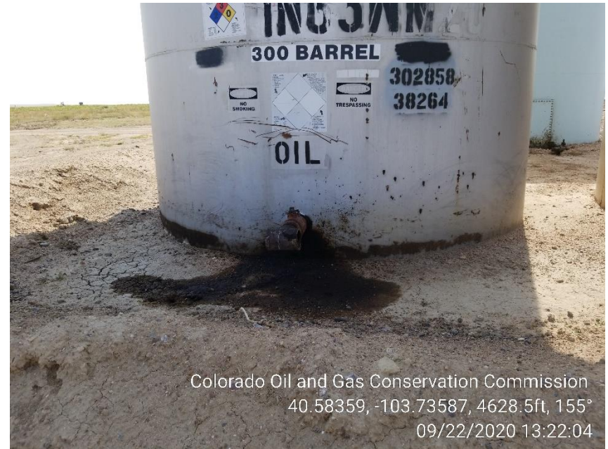
Photo 8 – Stained Soil at NE Tank
