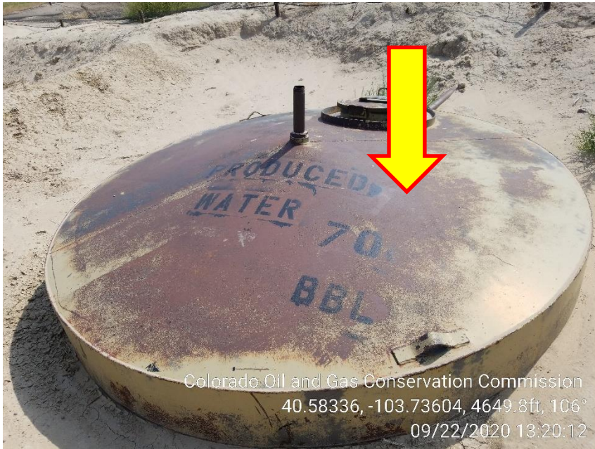
Photo 11 – Skim Tank missing NFPA Label
