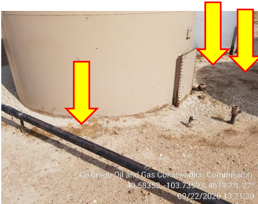
Photo 9 – Inside Tank Berm, Stained Soil. Risers now marked
