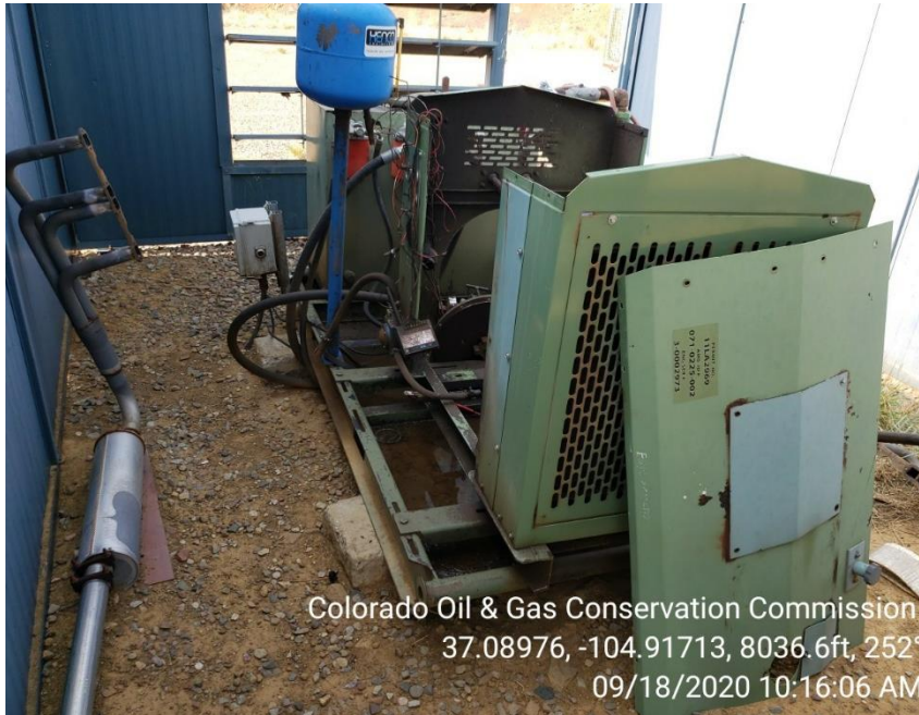
Photo 5 Engine skid no engine
