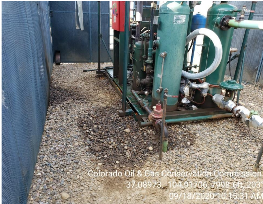
Photo 3 Stained oil at liquid ring
