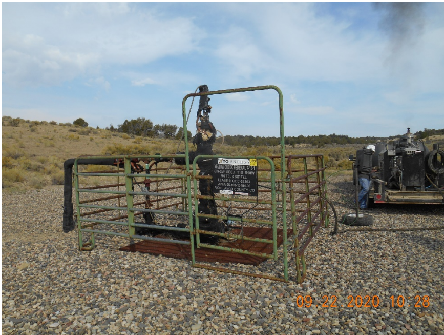
Injection wellhead
