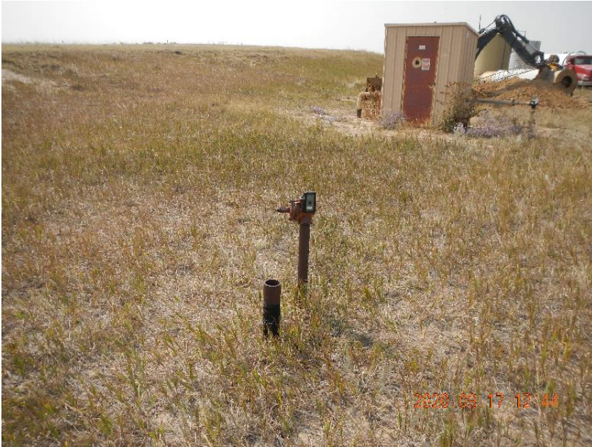
Photo 1: View of Trimble GPS unit at flow line risers E of gas meter run.
