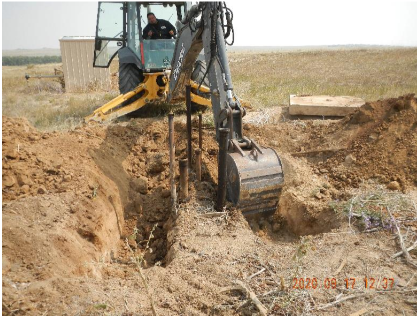
Photo 7: Excavating flow line risers at heater treater site.
