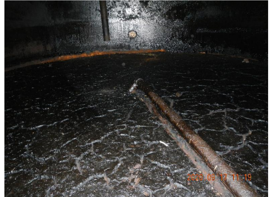
Photo 6: View inside unused tank after hatch removed.
