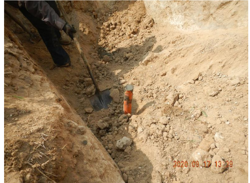
Photo 10: Cement plugging risers for abandonment.
