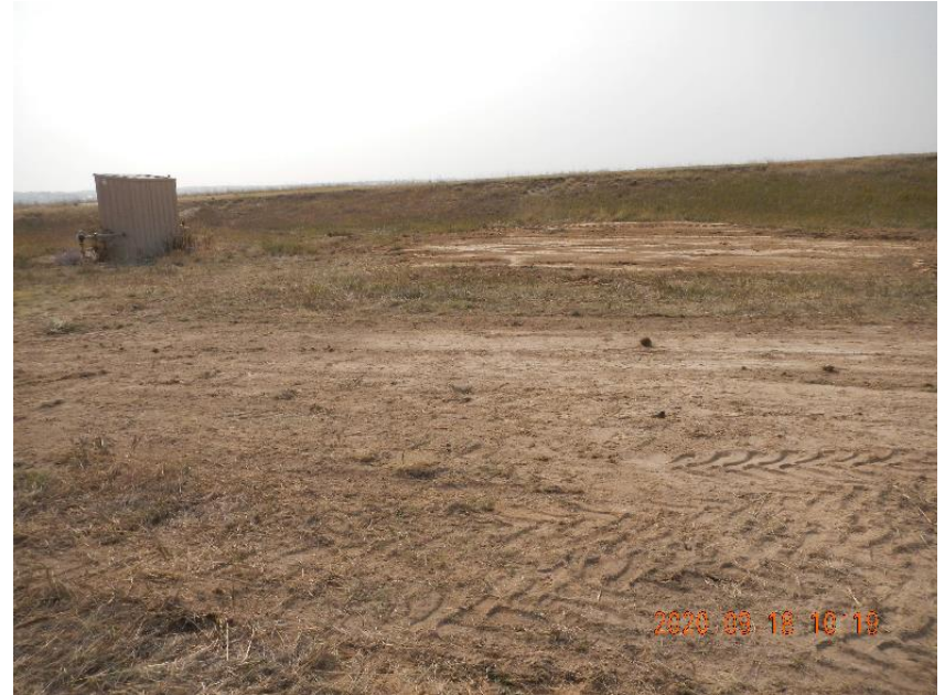
Photo 16: View of redressed excavation sites.
