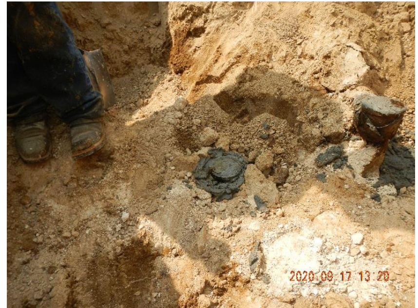
Photo 8: Cement plugging flow lines for abandonment.
