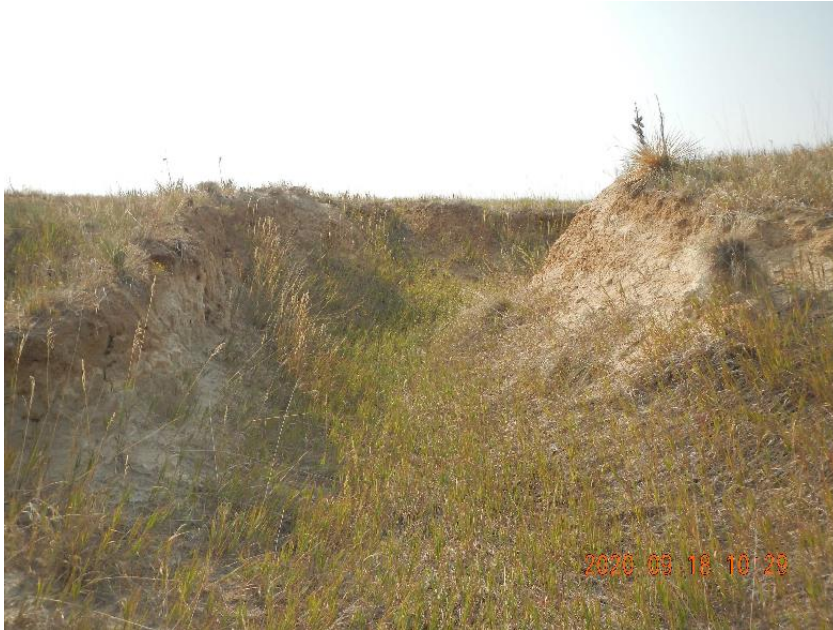
Photo 19: View from inside erosion gully looking up slope.
