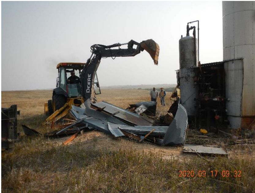
Photo 3: Tearing down heater treater shed.
