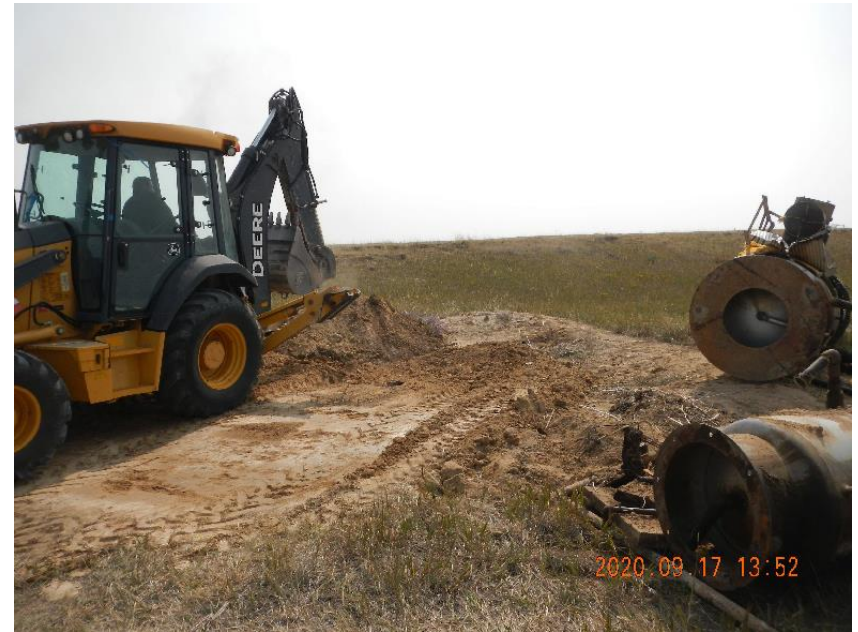
Photo 12: Backfilling excavation site at heater treater site.
