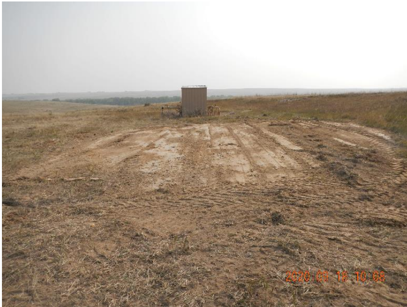
Photo 13: Backfilled and dressed excavation at heater treater site.
