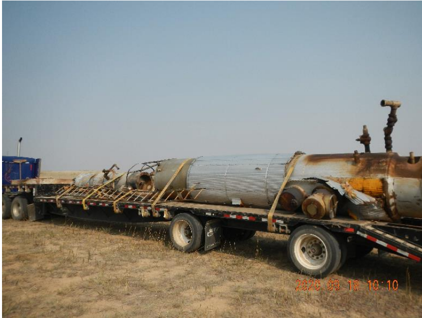
Photo 15: Treater, pipe, pipe fittings, and debris loaded for removal from location.
