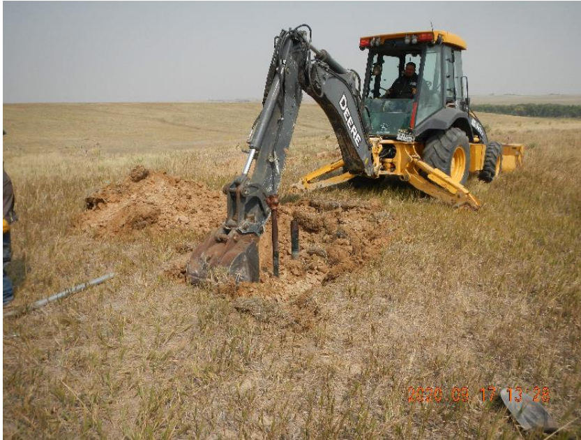
Photo 9: Excavating flow lines on E side of meter run shed.
