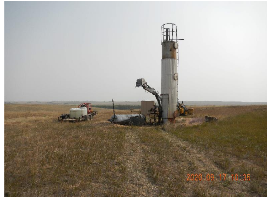
Photo 4: Laying down disconnected treaters for haul off and removal.
