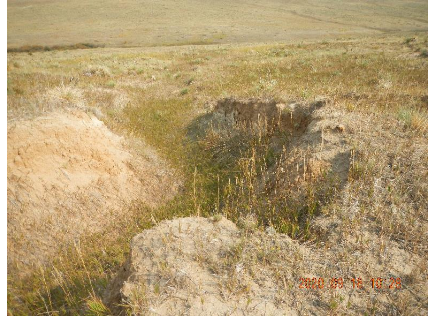
Photo 18: Additional view of erosion gully looking further down slope.
