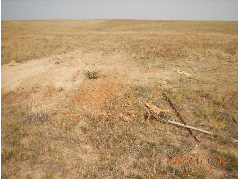
Photo 5: One of three anchors located and removed.
