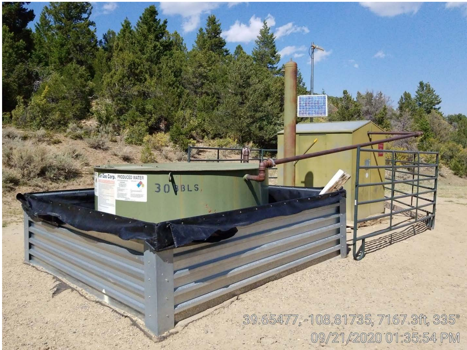
Photo 2. Tank & separator.
