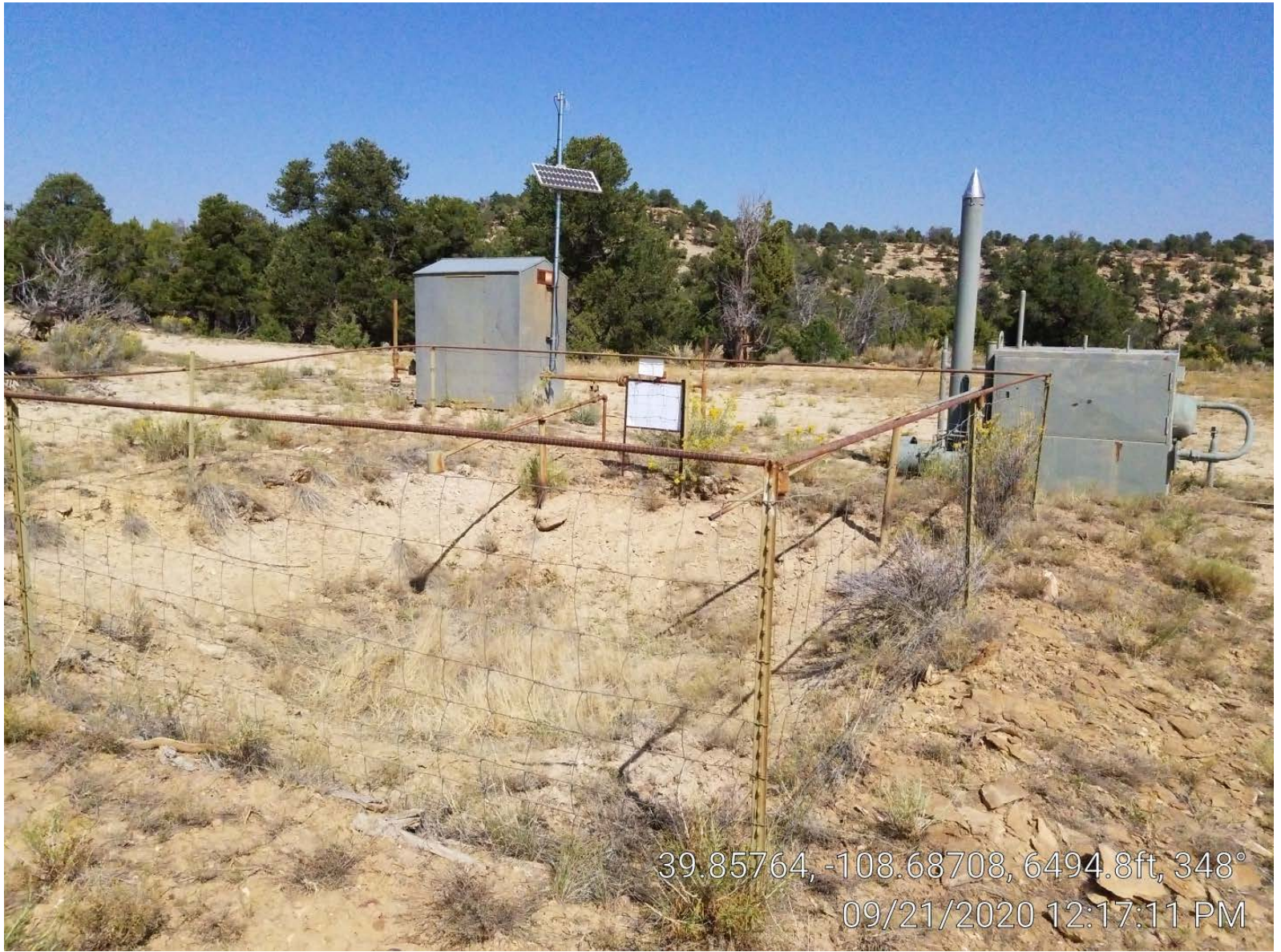
Photo 2. Pit, meter building, separator.
