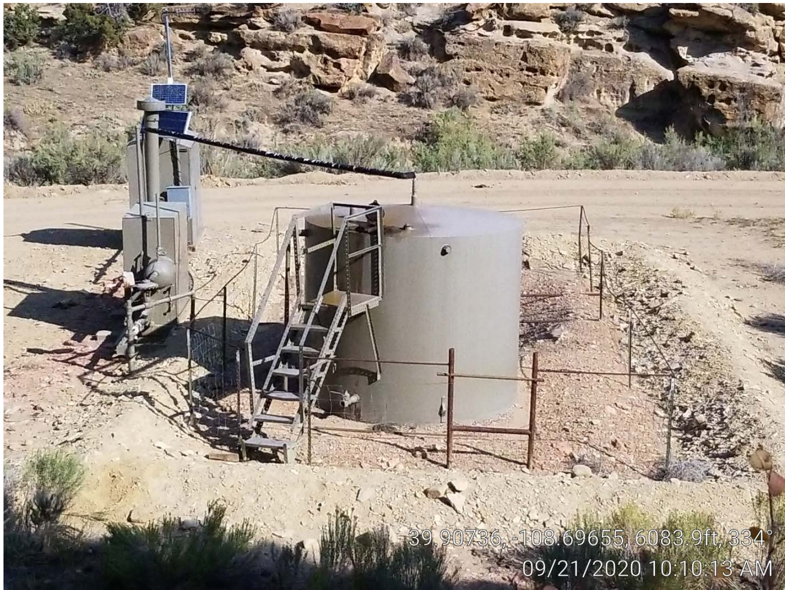
Photo 3. Tank, separator, meter building.
