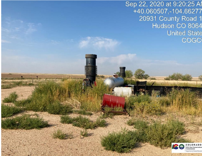
Pic 1 weeds / storage of equipment
