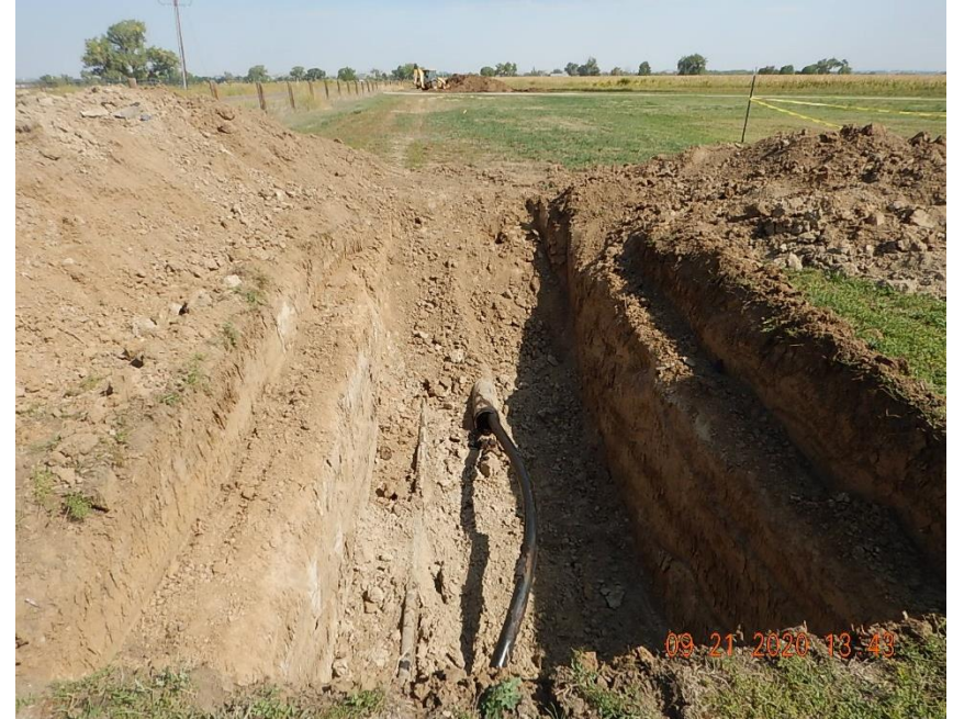
West bellhole excavation; 6" CS H Huett Consolidation OLF exposed and cut with 3" OD DR 11 HDPE pipe being slip lined through failed section of pipe. A 2" CS OLF is also exposed in the excavation.
