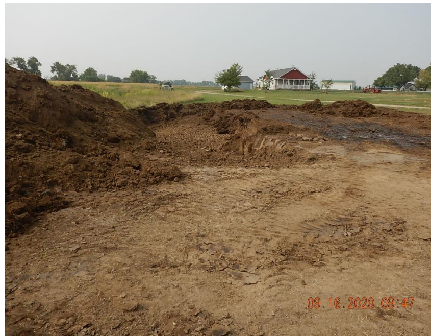
Closer view of area of release and hydrocarbon stained soils; view west.
