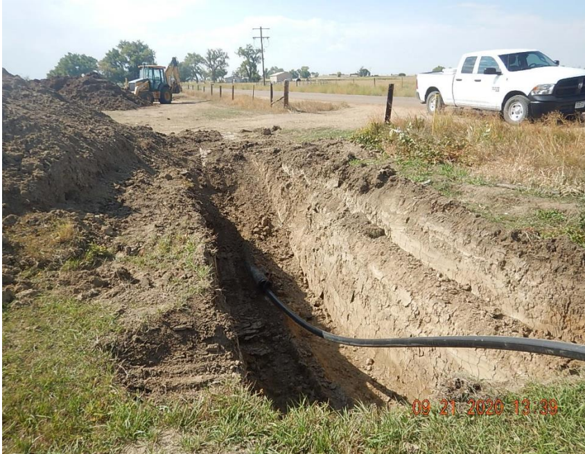
East bellhole excavation; 6" CS H Huett Consolidation OLF exposed and cut with 3" OD DR 11 HDPE pipe being slip lined through failed section of pipe.
