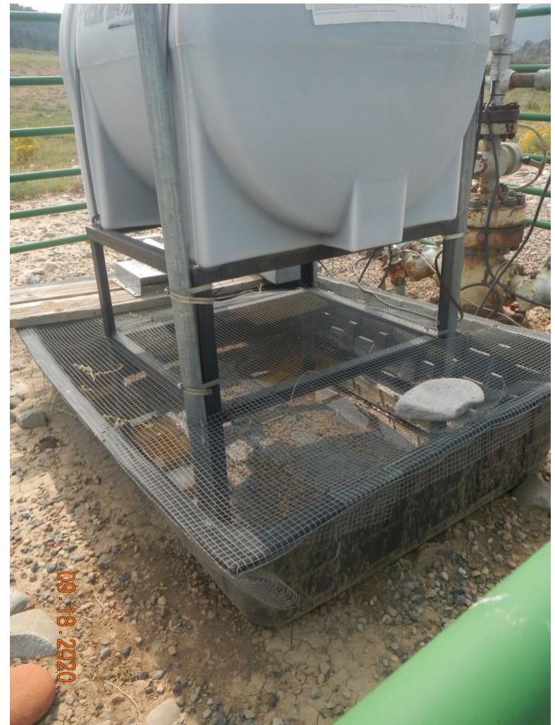
Photo#4: Secondary containment covered with screen
