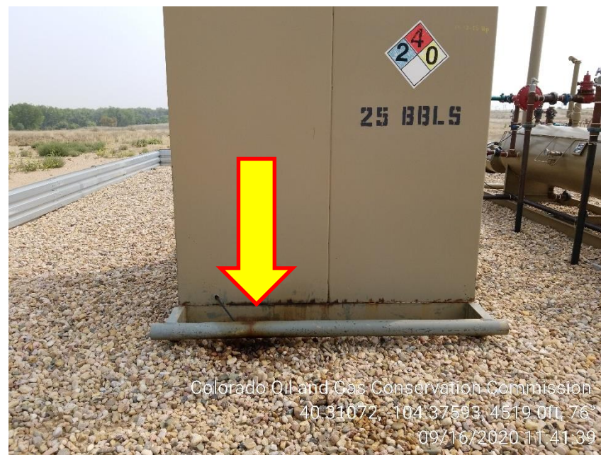
Photo 8 – Stained Soil at North Separator
