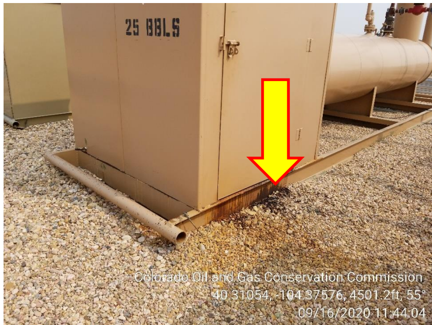
Photo 9 – Stained Soil at Middle Separator
