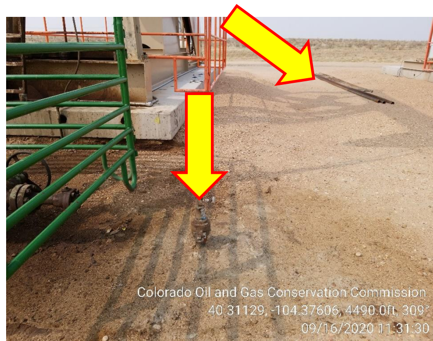
Photo 6 – 18-7-10 – Unmarked Riser, Stained Soil, Unused Tubing and Rods
