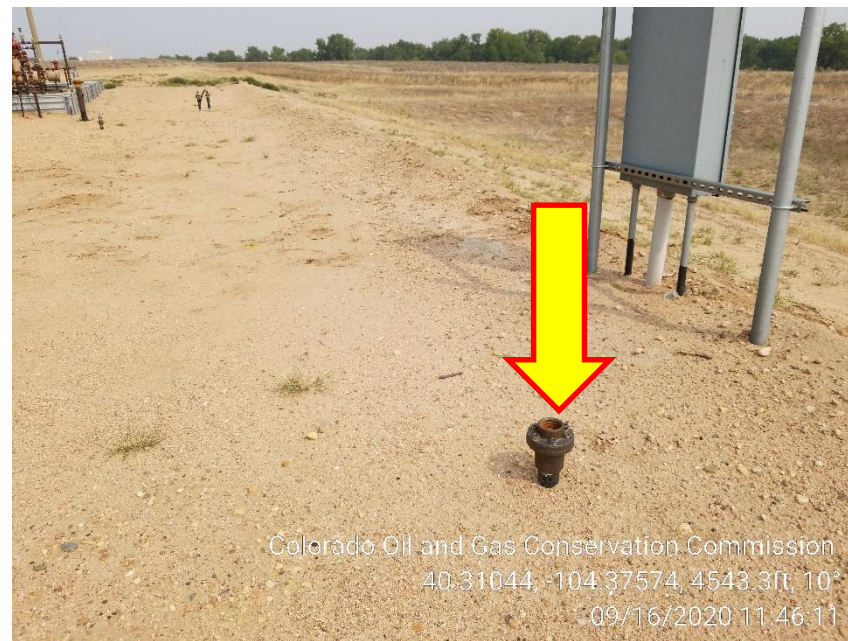
Photo 12 – Unmarked Riser
