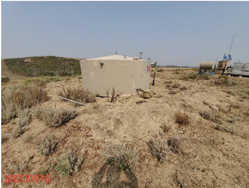
Photo 1: Photo of 200 bbl condensate tank on the southern end of the Location. Photo shows secondary containment remains out of compliance with Rule 906.d.(1); Vegetation remains established within BMP compromising the imperviability of the containment; BMP insufficient to contain contents of tank and sufficient freeboard to contain precipitation.
