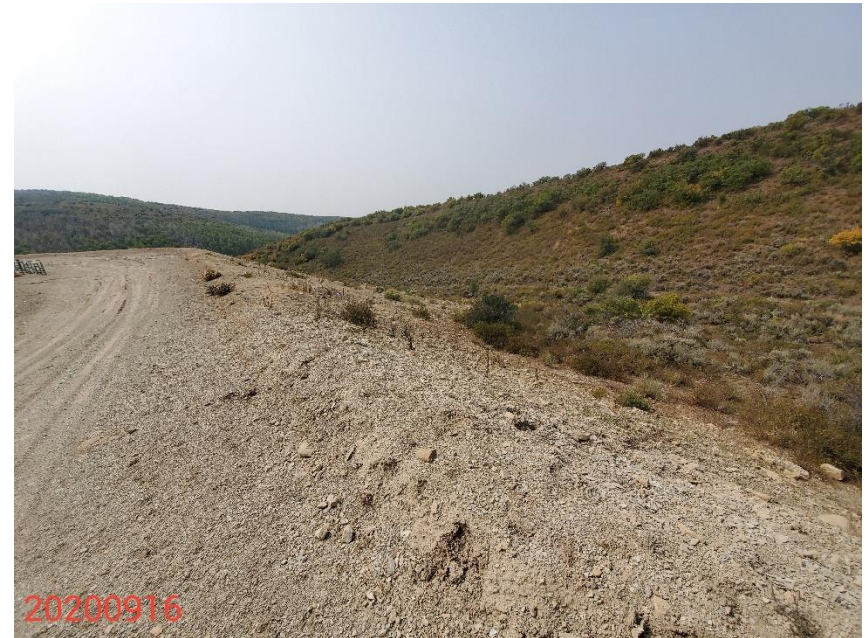
Photo 4: Photo taken from the west end of the Location, facing south. Photo shows BMPs on the Location remain missing or insufficient to stabilize soils on the slope. Photo also shows additional interim reclamation does not appear to have been conducted.
