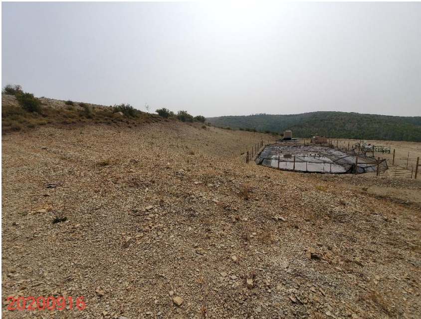
Photo 5: Photo taken from the east end of the Location, facing south. Photo shows BMPs on the Location remain missing or insufficient to stabilize soils on the slope. Photo also shows additional interim reclamation does not appear to have been conducted.
