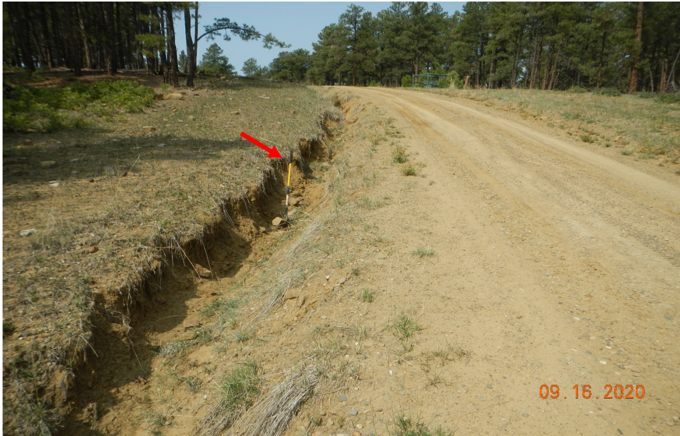
Photo 1. Facing northwest along the access road. Erosion has occurred along the road that needs to be repaired. Arrow points to 4.5 ft. shovel.
