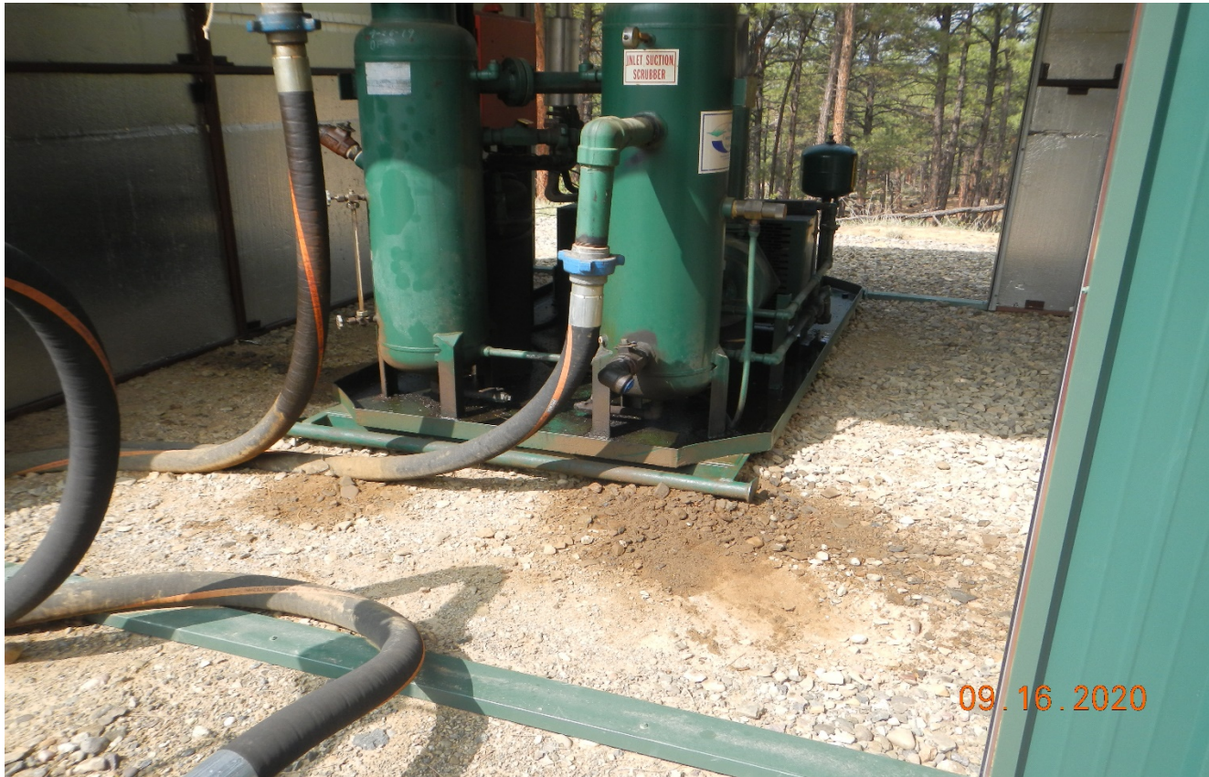
Photo 3. There is oil stained soil around the engine skid.
