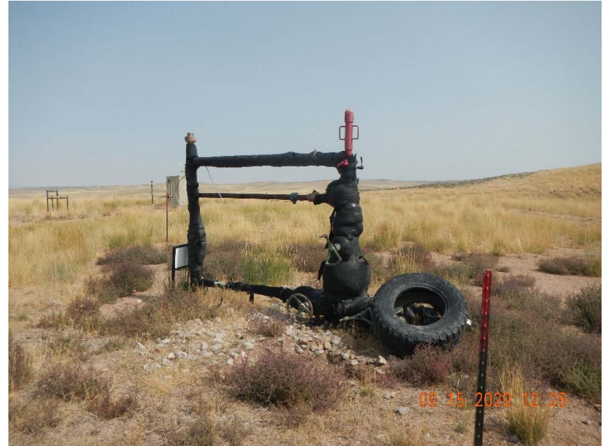
Photo 2. Annual weeds. Tire placed on wellhead.
