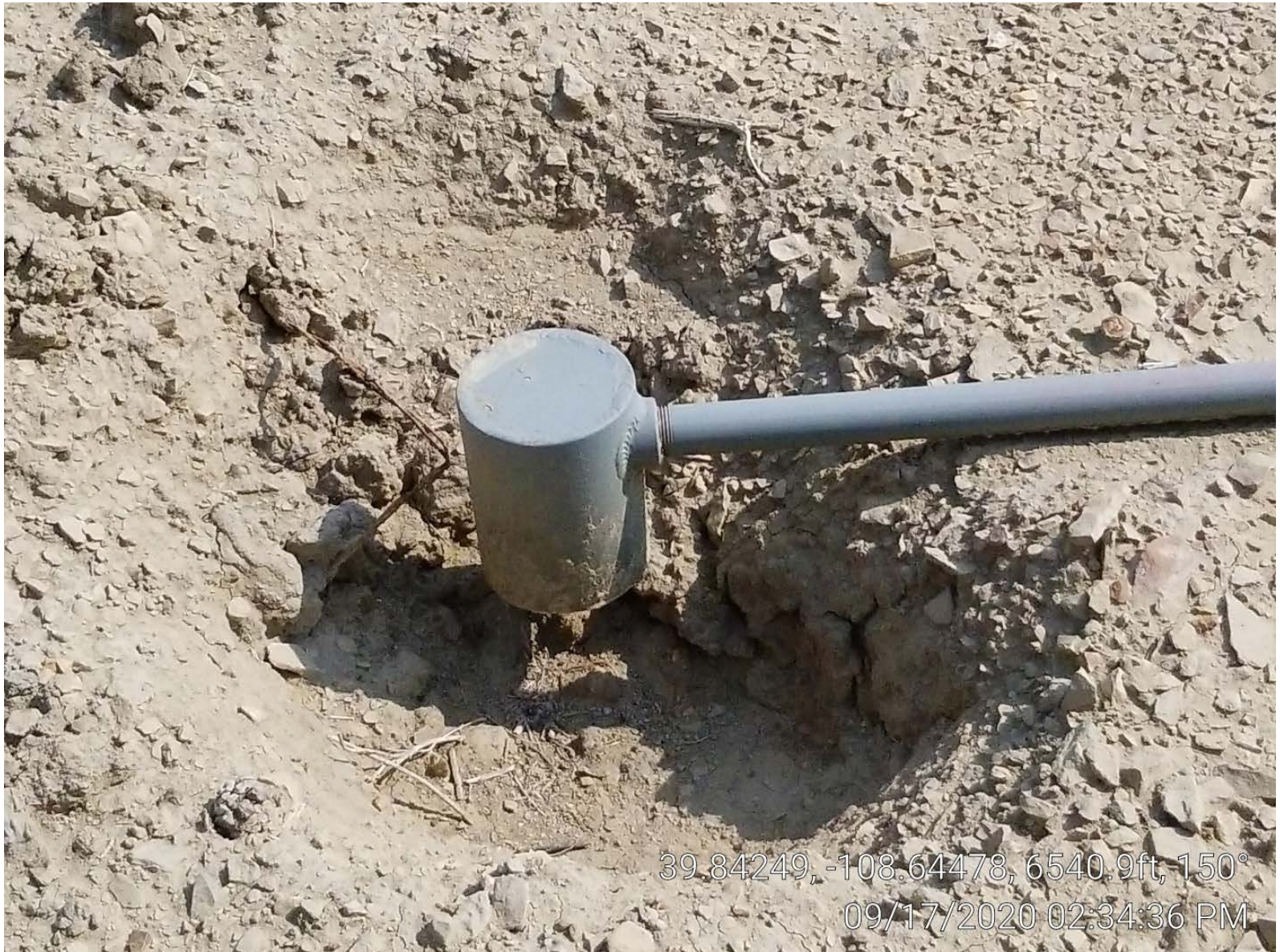
Photo 5. Pipe end within meter building pit.
