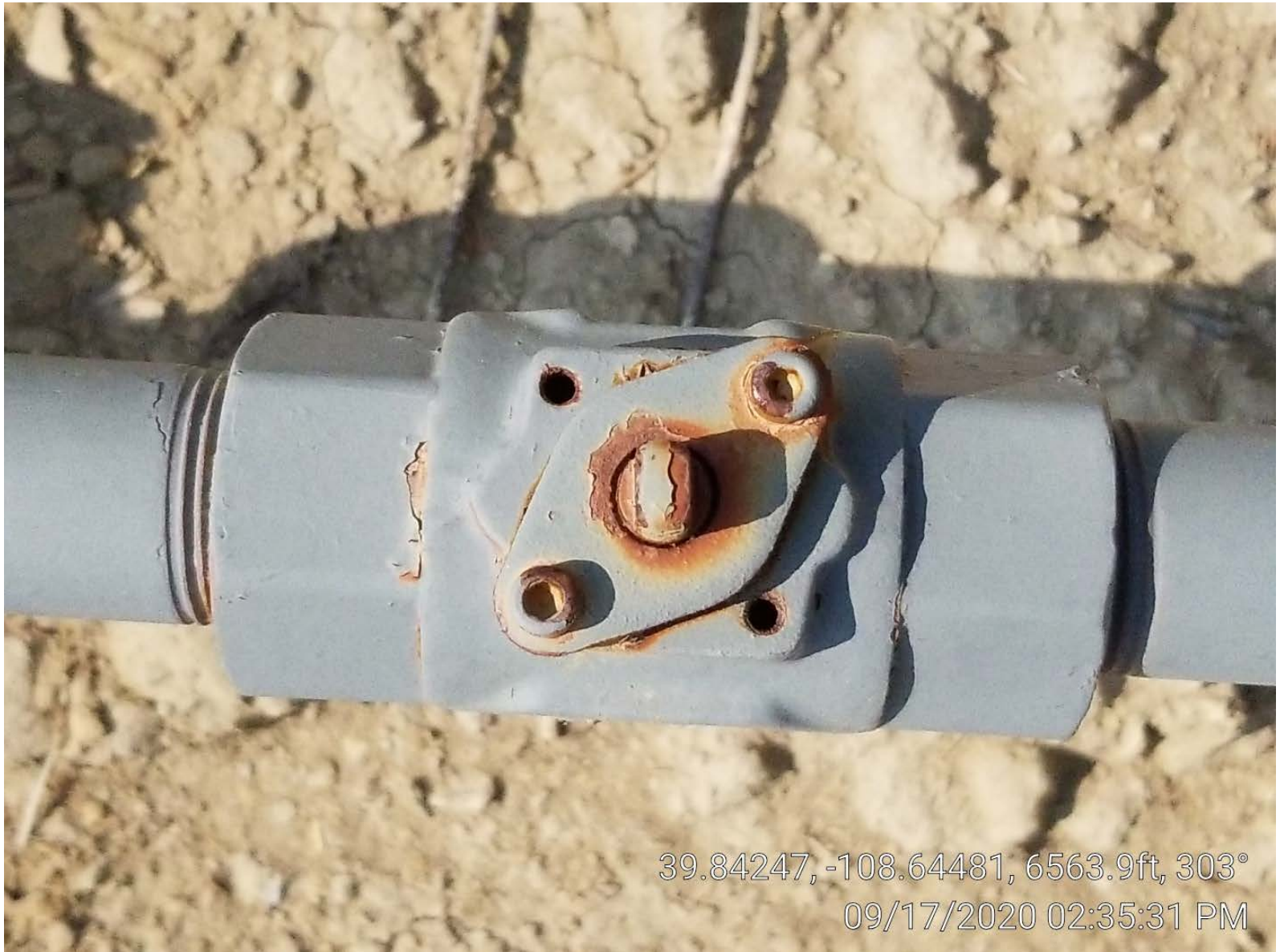
Photo 6. Meter building pit valve closed.
