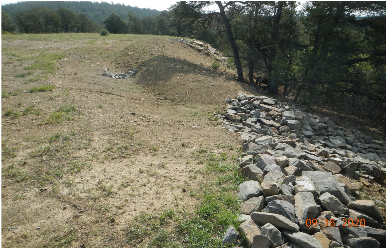
Photo 4. It appears there was recent work performed at the south side of the location with rock rip/rap installed.
