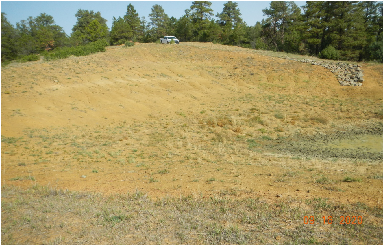
Photo 4. There is erosion along the cut slope of the pit which is not stabilized.
