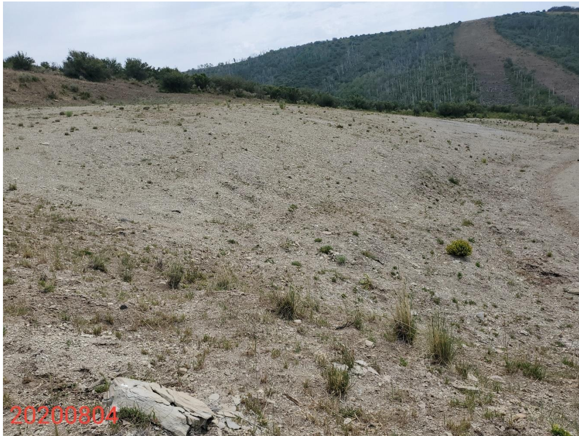
Photo 8.1 Photo copied from the 8/4/2020 inspection, taken from the northeast end of the Location, facing south. Photo shows interim areas. Soils at the surface appear to be subsoils; it does not appear that topsoil horizons were placed back to their relative original position.
