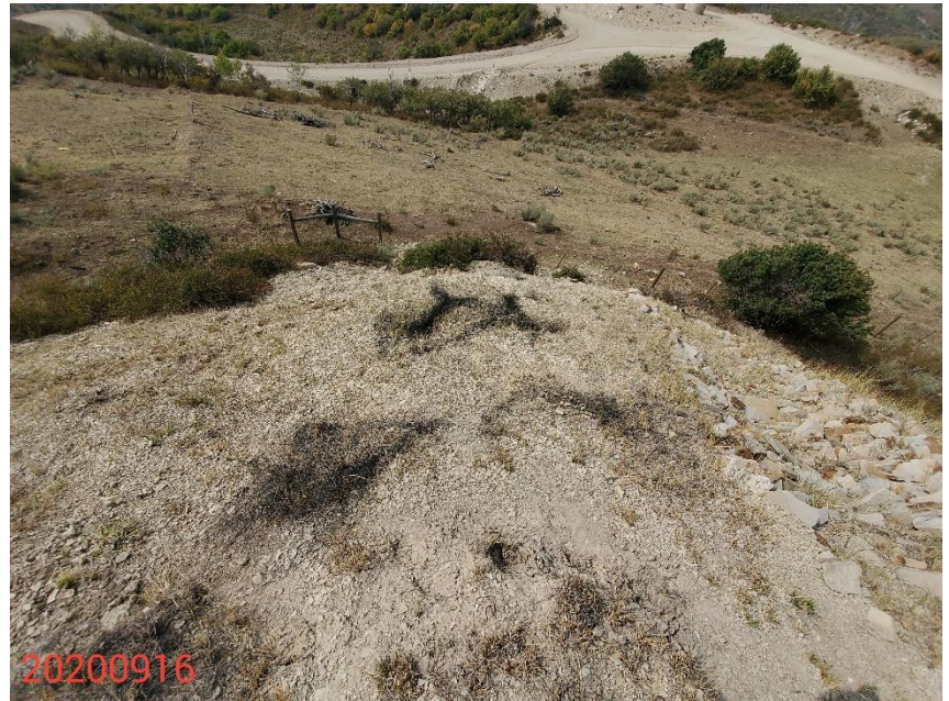
Photo 12: Continued from photo 11. Photo shows erosion net BMP remains in disrepair, and is considered Debris.
