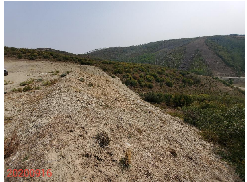
Photo 4: Photo taken from the southeast end of the Location, facing east. Photo shows areas of the Location, including fill slopes, that have not been recontoured/regraded or reclaimed to their original condition in accordance w/ 1003 rules. BMPs appear insufficient or missing to stabilize slopes.
