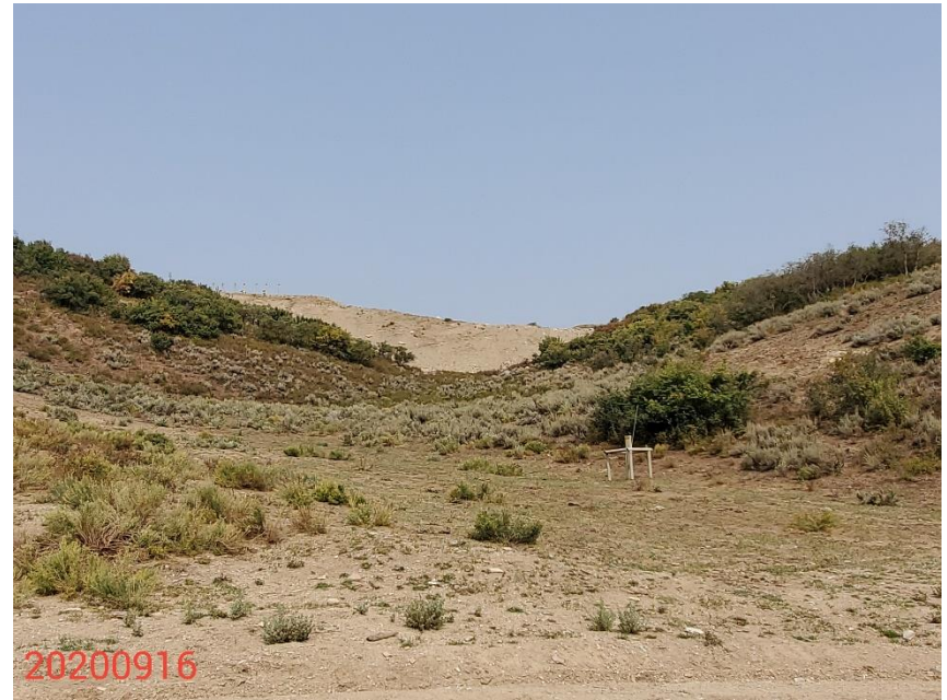
Photo 6: Photo taken from the south of the Location, facing north. Photo shows fill slopes that have not been recontoured/regraded or reclaimed to their original condition in accordance w/ 1003 rules.
