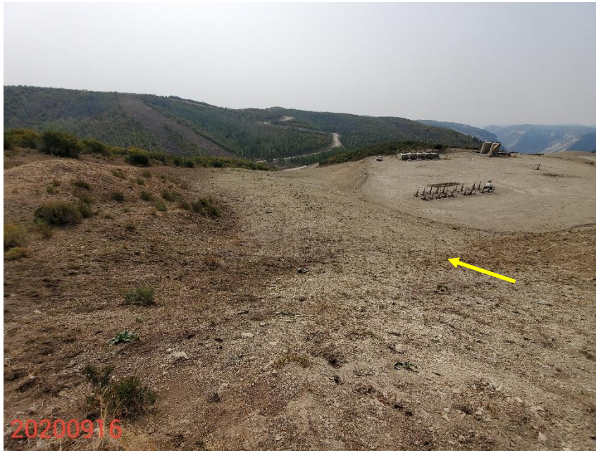
Photo 7: Photo taken from the east end of the Location, facing south. Photos 7-8 provide an overview of the Location from south to southwest. Photo also shows areas (left of arrow) that appear to be subsoils; it does not appear that topsoil horizons were placed back to their relative original position.
