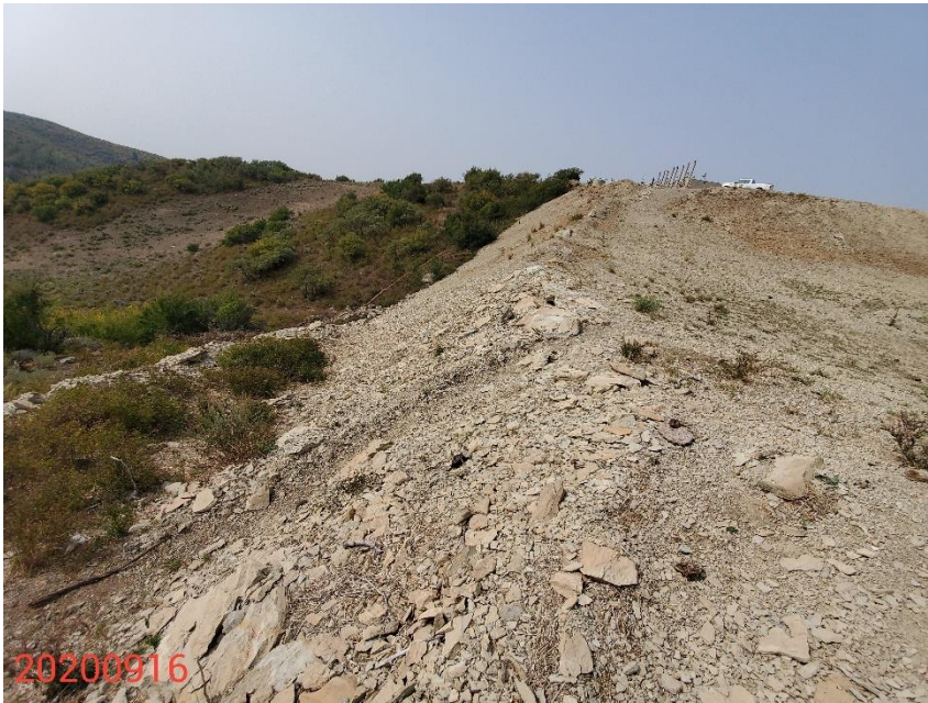
Photo 5: Photo taken from the southeast end of the Location, facing west. Photo shows areas of the Location, including fill slopes, that have not been recontoured/regraded or reclaimed to their original condition in accordance w/ 1003 rules. BMPs appear insufficient or missing to stabilize slopes. .
