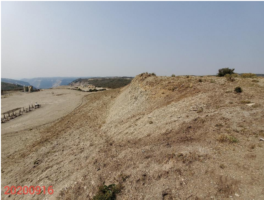
Photo 9: Photo taken from the east end of the Location, facing southwest. Photo shows cut slopes; interim areas have not been contoured/regraded and reclaimed to their original condition.
